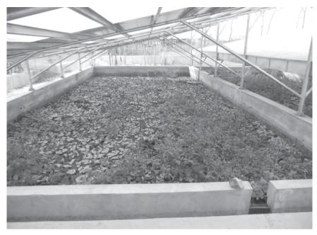
Photo 9.2 Drying bed cover arrangement, Jombang, Indonesia
