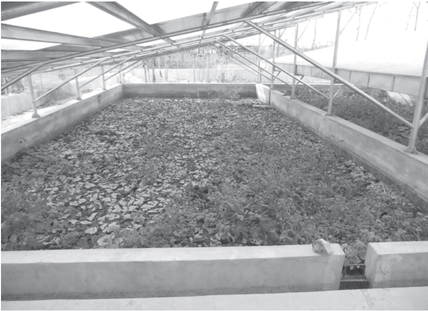
Photo 9.2 Drying bed cover arrangement, Jombang, Indonesia
