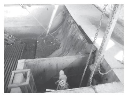
Photo 6.7 Run-down screen at Pula Gebang septage treatment plant
