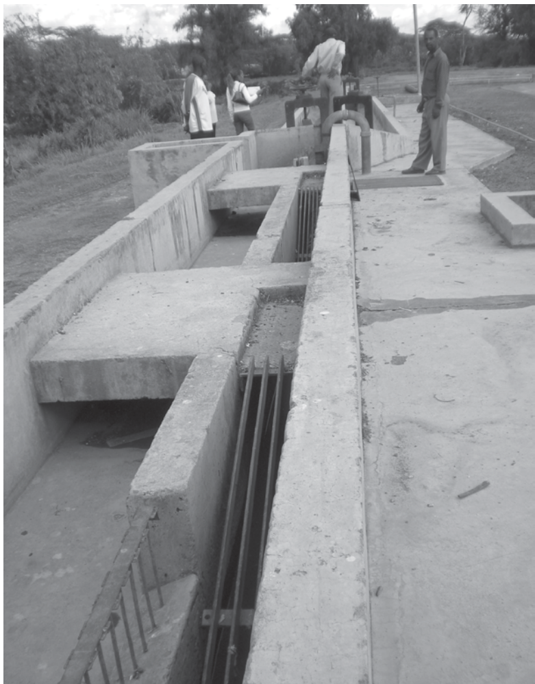
Photo 5.3 Inclined screen with operator access
