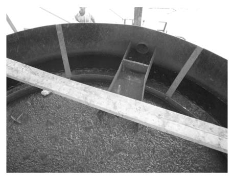
Photo 7.2 Arrangement for scum removal, Sittwe hopper-bottomed tank
