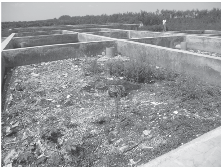
Photo 5.1 Sludge management problems in anaerobic pond, Tegal, Indonesia (note the lack of provision for operator access to the tanks)
