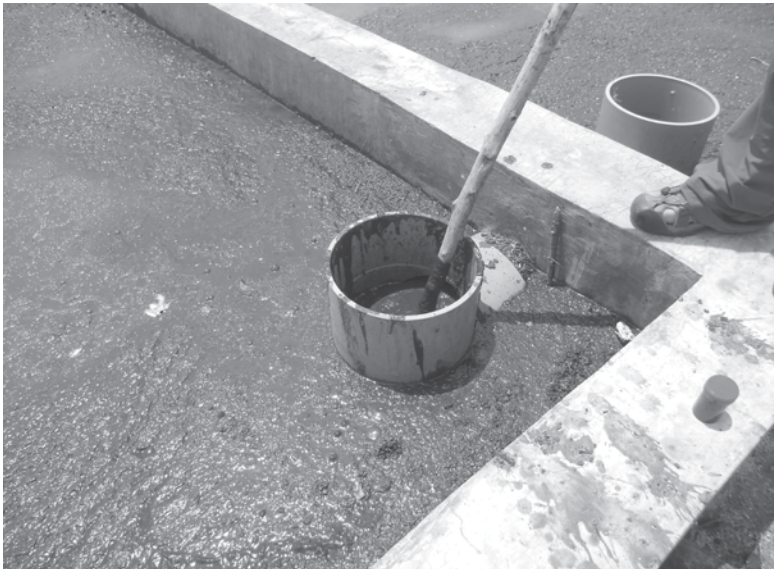
Photo 5.4 Blocked connection pipework
