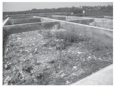
**Photo 5.1** Sludge management problems in anaerobic pond, Tegal, Indonesia (note the lack of provision for operator access to the tanks)
