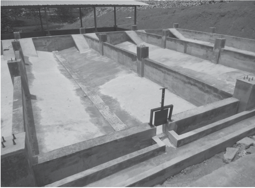
Photo 9.1 Drying beds under construction
