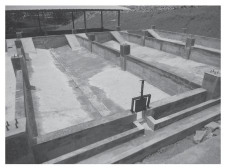
Photo 9.1 Drying beds under construction
