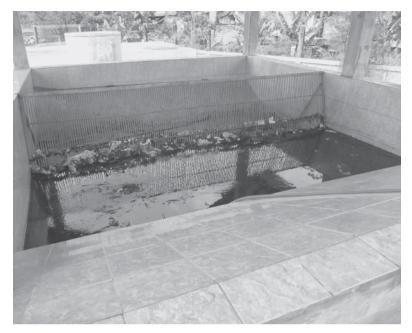
**Photo 5.2** Vertical screen with no operator access
