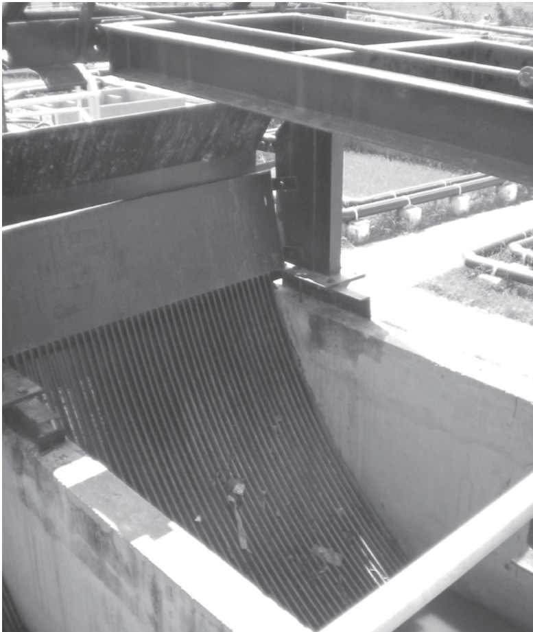
Photo 6.6 Curved screen with rotating raking mechanism
