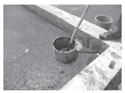
Photo 5.4 Blocked connection pipework
