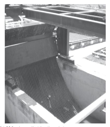
Photo 6.6 Curved screen with rotating raking mechanism
