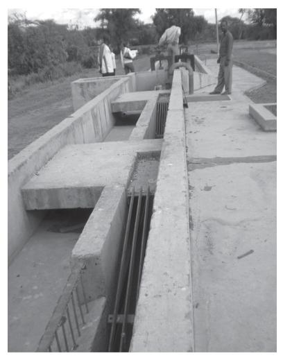
Photo 5.3 Inclined screen with operator access
