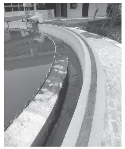
Photo 5.5 Unbalanced flow resulting from poorly levelled weir
