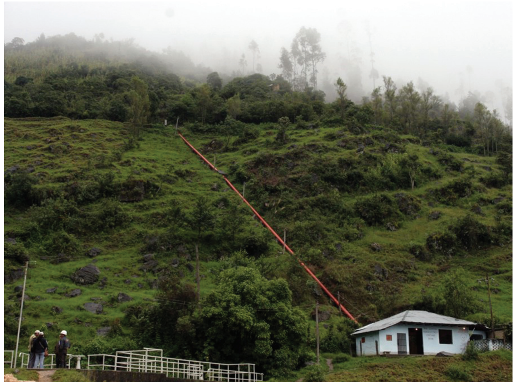
Power house of the Conchán micro-hydro, Cajamarca, Peru
