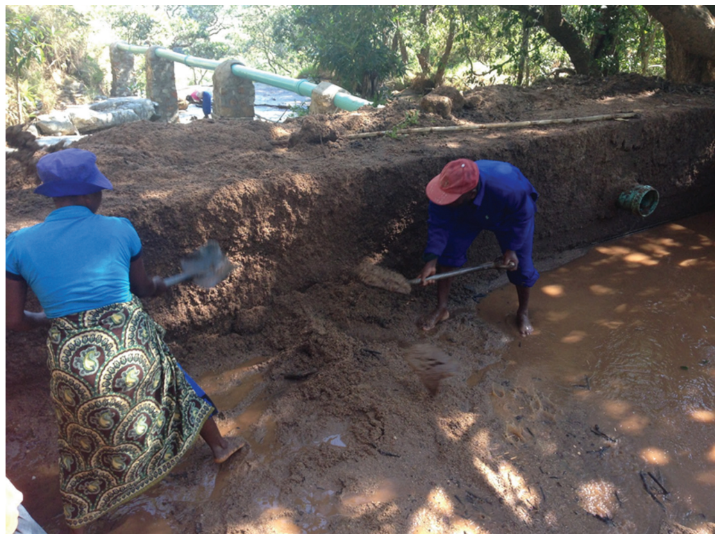
Clearing silt from the weir at Ngarura, Zimbabwe
