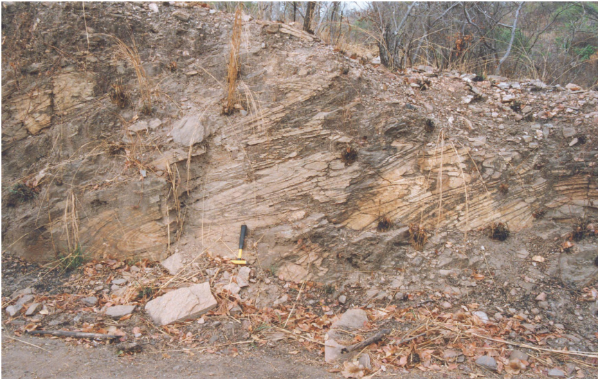
A46. Folded schistose pelites and meta-sandstones in a road cutting in Zambia. BGS, © NERC 2000.
