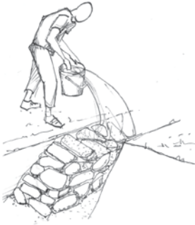
Figure 95: Interrupted foundation work must have staggered and rough ends. Keep fresh foundations moist.
