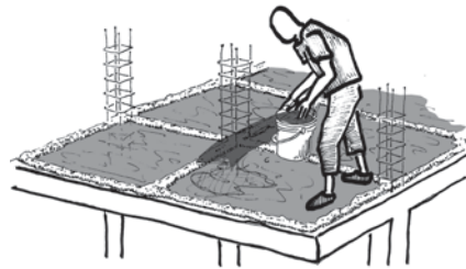
Figure 191: Keep the slab under water for two weeks
