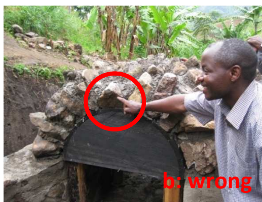
Fig. 40: a: Stones are tightly put together. They should act as a wedge with the narrow base pointing downwards. Fig 40 b: The keystone is wrongly placed. As the large base is at the bottom, the stone will fall out over time.
