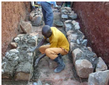
Abutment construction
