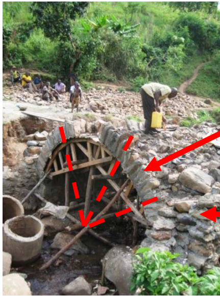
Fig. 24: Different positioning of stones in the structure
