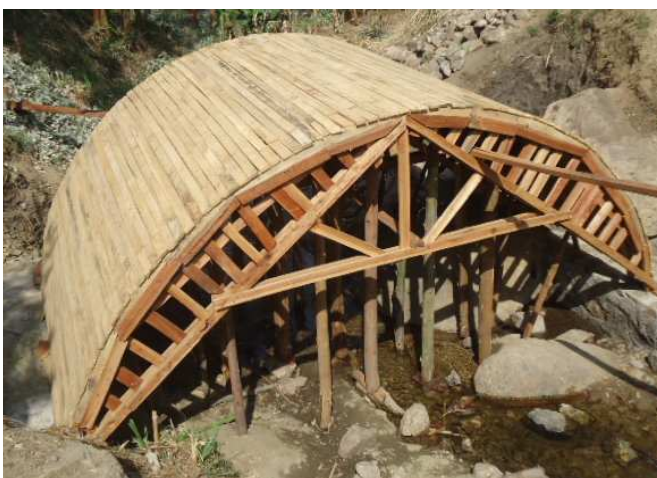
Fig. 25: Each truss of the form work consists of 2 pre-fabricated quarter circles that are assembled at site.
