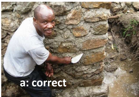
Fig. 23 a: The quality of stone masonry is essential. A good bond of stones and tight gap filling will provide for a strong abutment. In addition, at the river corners dents are left for a good link with the wing-walls. Fig. 23 b: Extremely poor masonry works – no bond at all, plenty of gaps between the stones, no embedding of stones with mortar. Sections like those need to be demolished immediately and the mason replaced.
