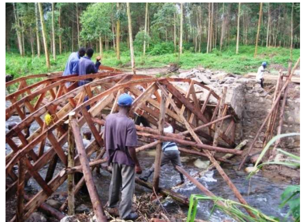
Fig 29: five trusses are required for a standard width of 3.6 m. The trusses are supported by struts.
