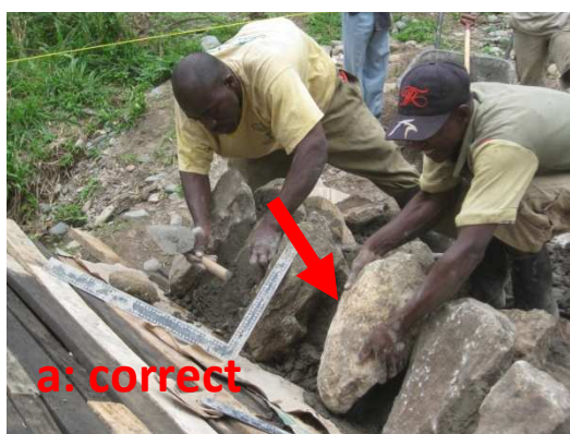
Fig. 40: a: Stones are tightly put together. They should act as a wedge with the narrow base pointing downwards. Fig 40 b: The keystone is wrongly placed. As the large base is at the bottom, the stone will fall out over time.
