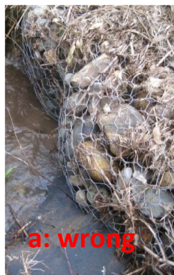
Fig 43: If not properly installed, gabions often collapse fast (a). This example started sagging after the first flood and had to be redone. Before the gabions are placed at the river banks, large stones will be rammed in as support basis to avoid early scoring under the gabion. The stones are carefully placed in the cage to avoid damaging the galvanized coating. The craftsmen will look for a good bond between the stones (b). The stone volume in the cage is 100% self supporting. There is no pressure of the stones on the cage. All cavities are filled with small stones and river sand. The gabions are filled in such way, that if walking on them, the stones should not move (c). Half way the filling, wires are tied to across the cage to reinforce the gabion
