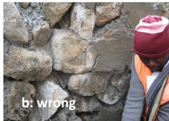
Fig. 23 a: The quality of stone masonry is essential. A good bond of stones and tight gap filling will provide for a strong abutment. In addition, at the river corners dents are left for a good link with the wing-walls. Fig. 23 b: Extremely poor masonry works – no bond at all, plenty of gaps between the stones, no embedding of stones with mortar. Sections like those need to be demolished immediately and the mason replaced.
