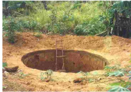
Figure 3: Pit for the tank construction
