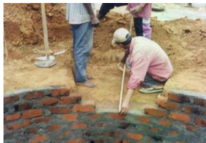
Figure 6: Measurement taken for the inlet construction
