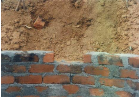
Figure 10: Outlet of the tank
