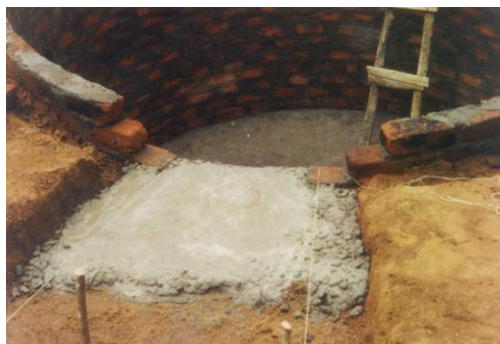
Figure 7: Concrete base for the inlet construction
