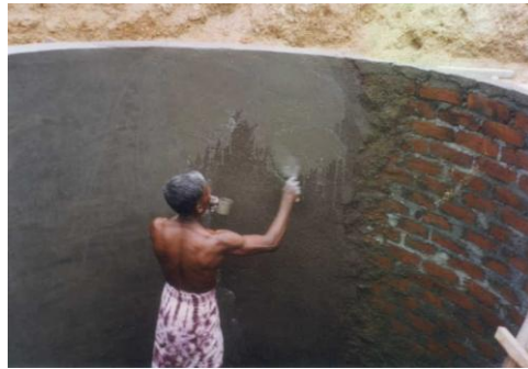
Figure 12: Plastering the tank
