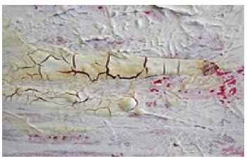
For blistering, flaking, peeling and cracking; identify & eliminate source/s of dampness. Remove loose paint, ensure surface is free of grease, and allow to dry. Apply primer coat and repaint following manufacturer's instructions.
