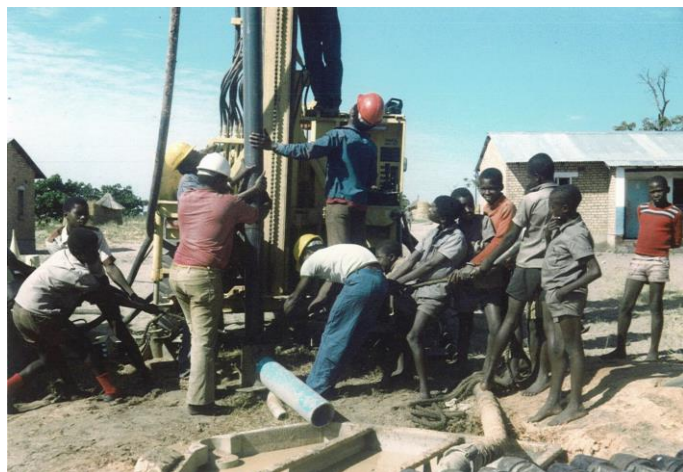
Figure 4: Installation of Casing
