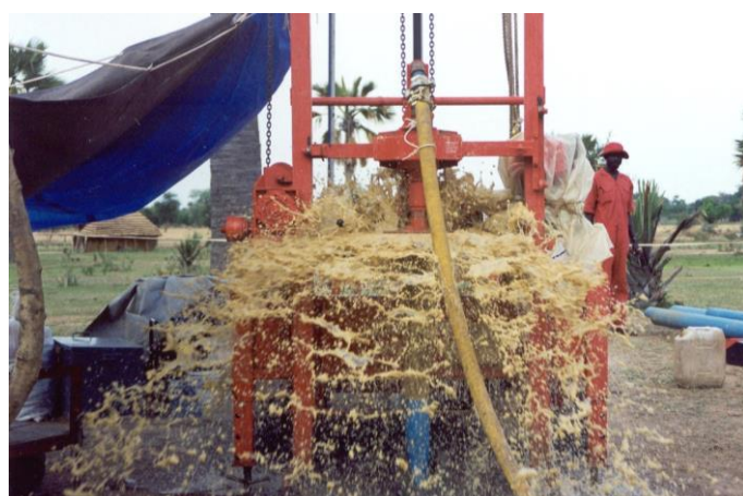
Figure 5: Well Development using Compressed Air
