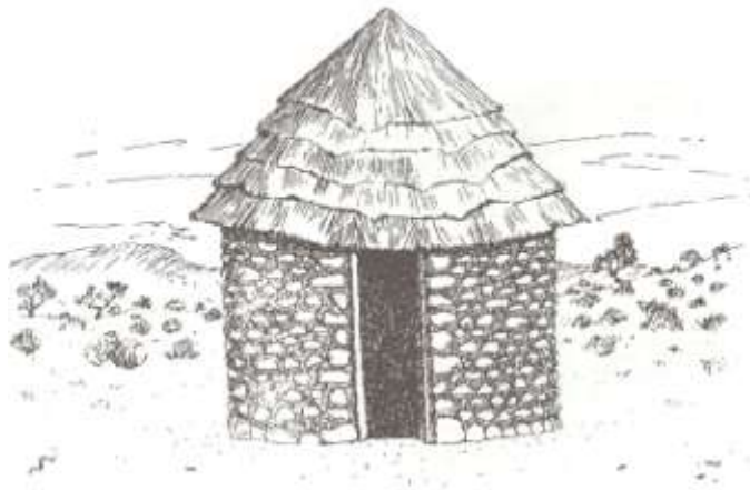
Figure 1: A rondavel built of earth and stone.
