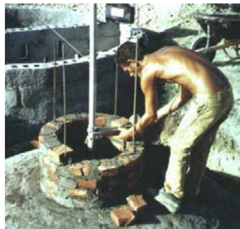
Figure 16: Construction of the digester neck with steel reinforcement Photo: Krämer (TBW)
