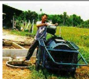
Figure 42: Drying of digested sludge and sludge disposal in Thailand
