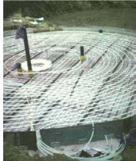
Figure 31: Heating system for a biodigester under construction (Germany)
