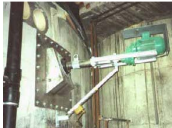
Figure 19: Stirring device for a european biodigester
