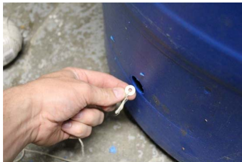
Figure 1. Drill a 3/4" hole in the barrel about 1" from the bottom (if no outlet).
