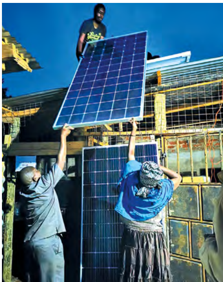
Figure 6.8 PV modules installation ( Solar Cooling Engineering ).
