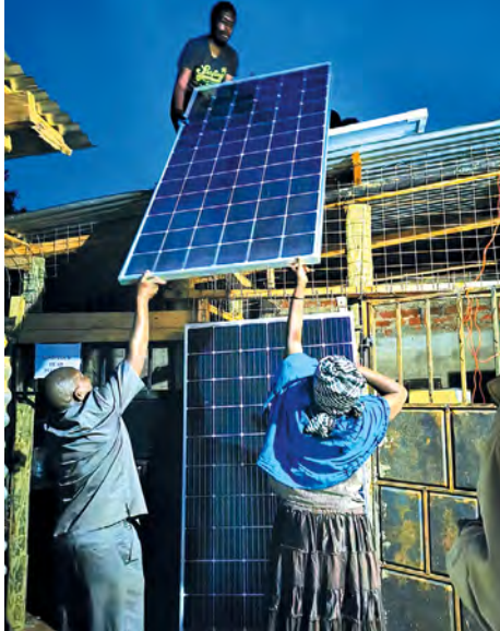
Figure 6.8 PV modules installation ( Solar Cooling Engineering ).
