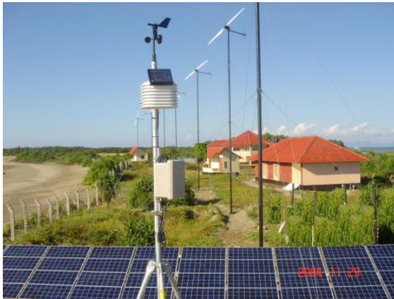
Wind, 5kWp -Solar, 5kWp Hybrid System at St. Martins Island, Cox's Bazar, Bay of Bengal, Bangladesh
