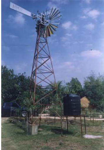
Water Pumping Windmill, designed by LGED
