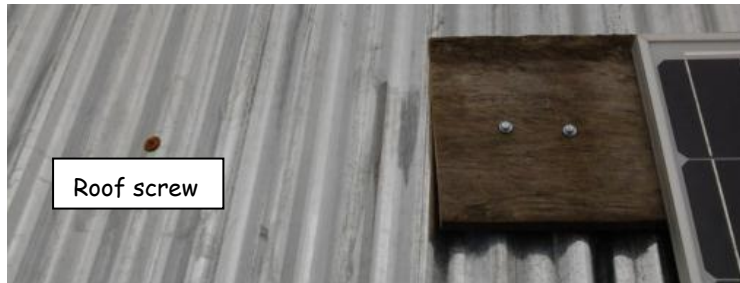
The roof screws serve as a guide.
