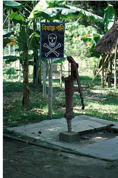
Figure 1: An arsenic poisoned well in Bangladesh. When arsenic is found to be above the limit the well is painted red to indicate it is not suitable for drinking. Wells that are safe are painted green. Photo: Practical Action / Zul Mukhida.
