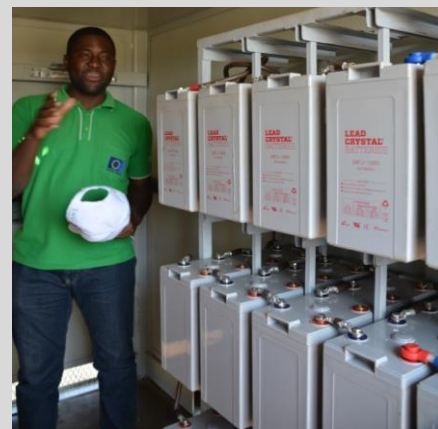
Figure 3: Mashaba clinic and mini-grid battery bank
