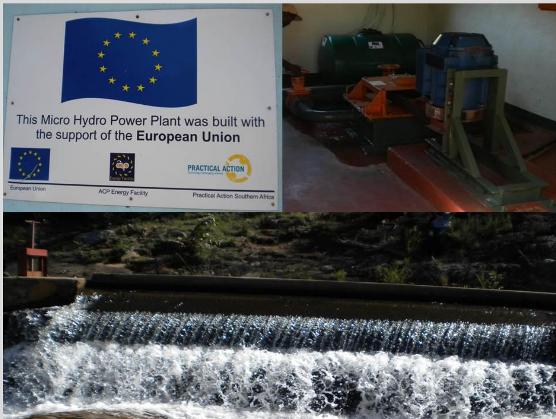
Figure 4: Chipendeke mini-hydro power plant
