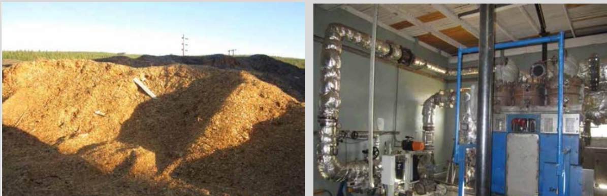
Figure 5: Wood shaving waste heaps and steam generation plant
