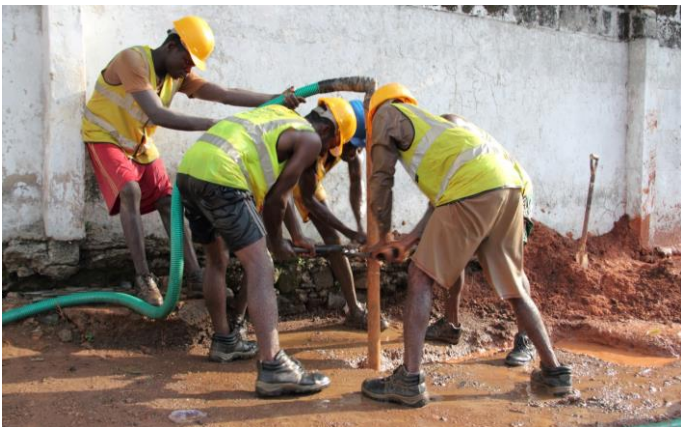
Figure 2: Drill Crew undertaking well jetting in Nigeria
