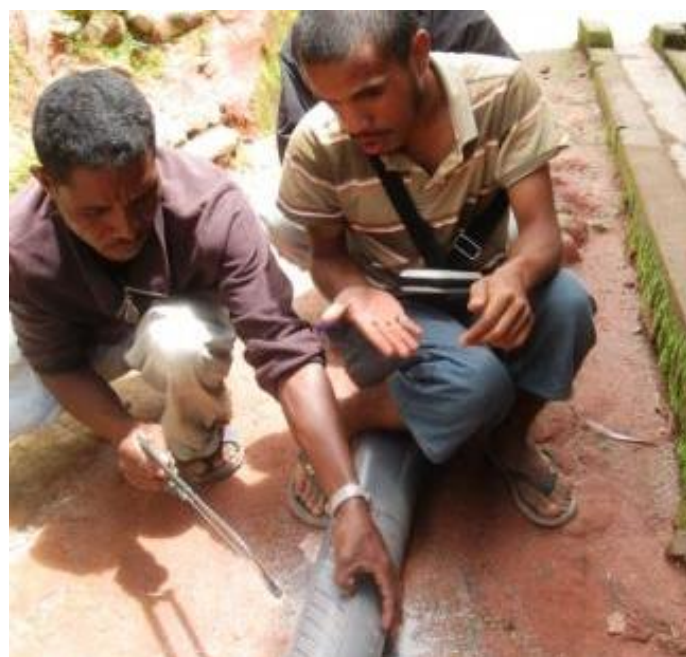
Figure 9: Masons cut slots in casing in Madagascar
