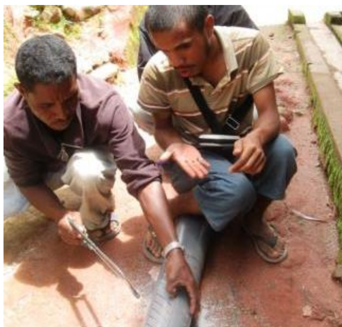
Figure 9: Masons cut slots in casing in Madagascar
