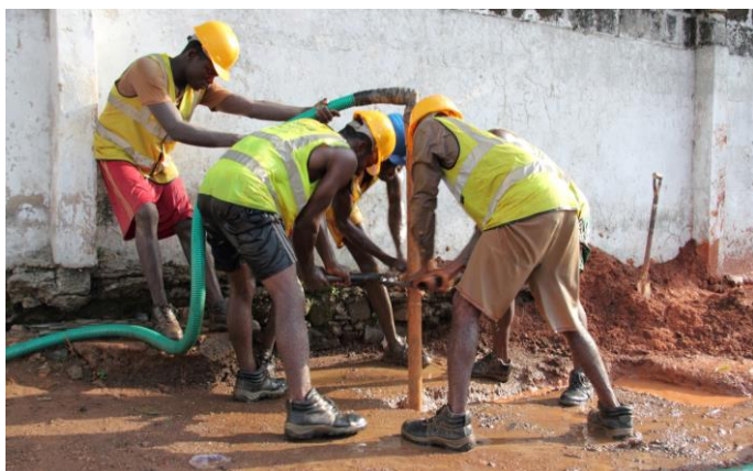
Figure 2: Drill Crew undertaking well jetting in Nigeria
