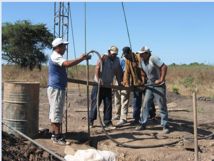
Figure (above) EMAS Percussion-Jetting-Rotation manual drilling, Trinidad, Beni region (Source Mike MacCarthy)
