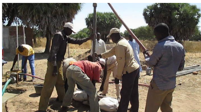
Figure 13: Jetting a household supply in Clesoum, N’Djamena
