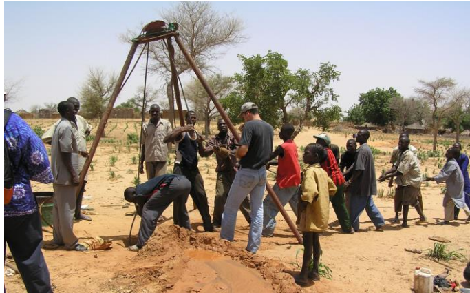
Figure 3: Percussion Drilling in Niger (Source: Richard Carter)
