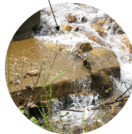
Figure 3: Reinforced concrete intake structure at Chontabamba – despite being only a few years old, there is already significant concrete and scour damage. Photos: Sakthy Selvakurmaran.
