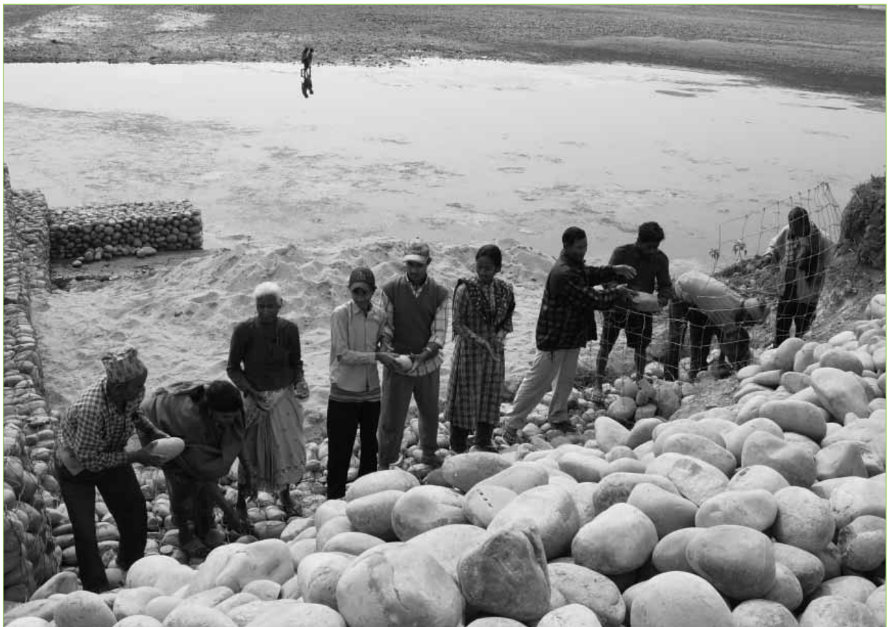
Gabion construction for flood protection in Kolhuwa, Nepal
