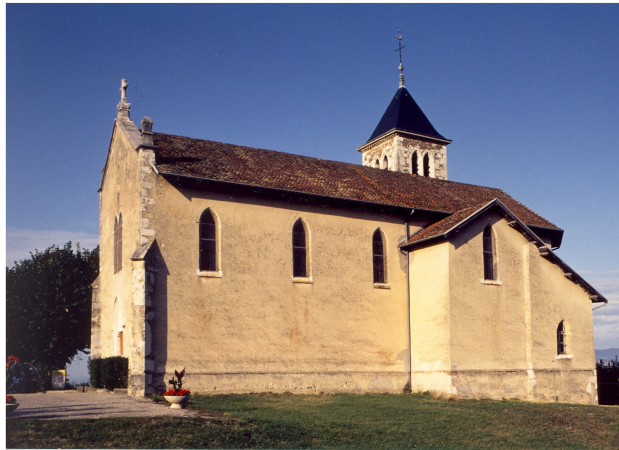
Figure 3: Church built in pisé (rammed earth) at Charancieu in the Dauphiné region of France. Photo: CRATerre/EAG
