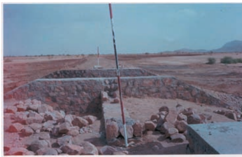
Turra dam: an upper view of the embankment
