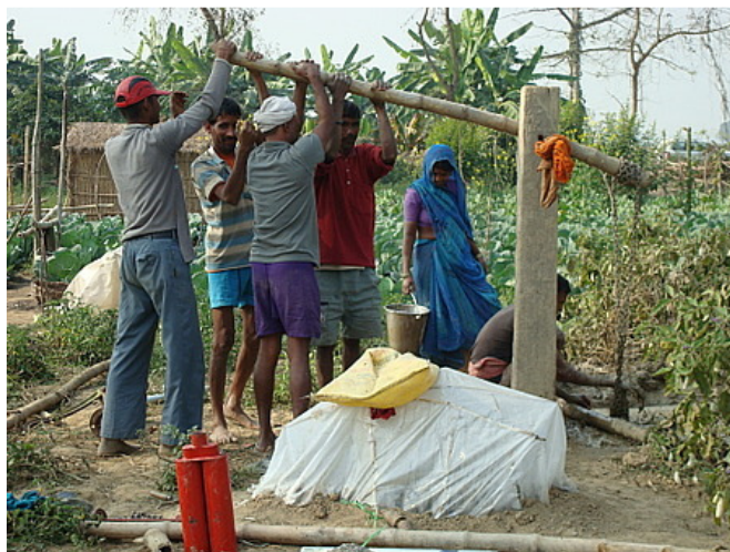
Figure 7: Farmers, from Mainhiya Village Development Committee, installing a treadle pump for irrigation. Photo: Practical Action Nepal / Matrika Sharma.
