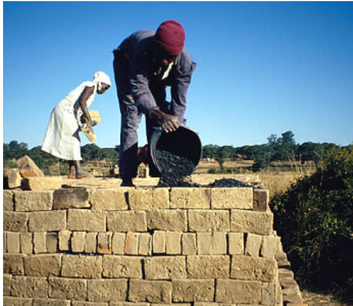
Figure 1: Boiler waste is sieved and used as a fuel for firing brick clamp kilns at Kurewasekwa Cooperative in Epworth, Harare. Photo: Practical Action / T. Schilderman
