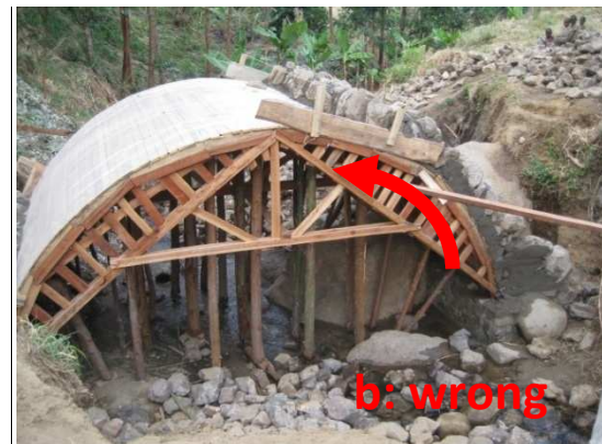
Fig. 41: For stability reasons, the bridge is built symmetrically, stepwise from both sides at the same time (a). It is dangerous to construct only one side first (b). The structure is not secure until the arch is closed in the middle.
