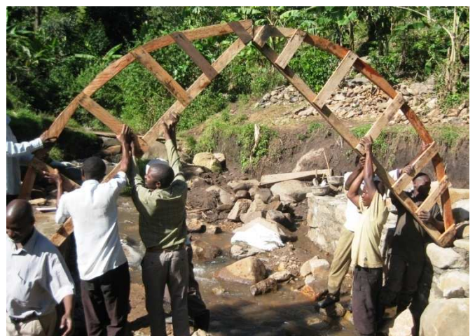
Fig. 25: Each truss of the form work consists of 2 pre-fabricated quarter circles that are assembled at site.
