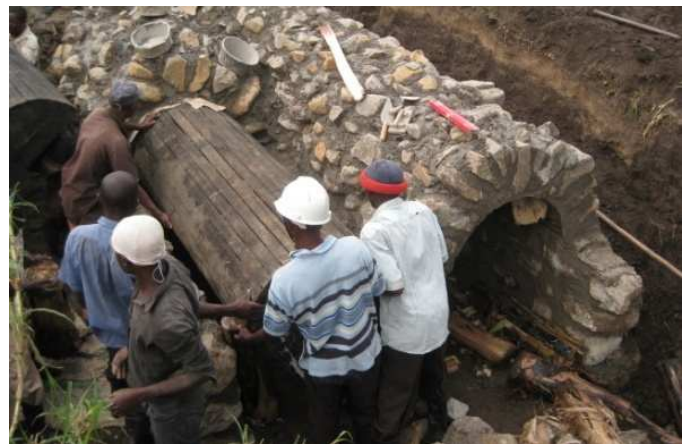
Fig. 33: The moulds for culverts are standard (here 80 cm diameter and 2 metres long). They can be re-used many times. The culvert size can be adjusted in function of the site conditions (banks, water flow) by increasing the abutment height or having multiple structures.
