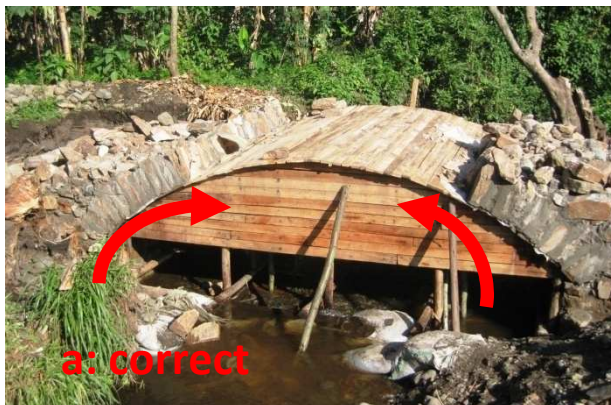
Fig. 41: For stability reasons, the bridge is built symmetrically, stepwise from both sides at the same time (a). It is dangerous to construct only one side first (b). The structure is not secure until the arch is closed in the middle.
