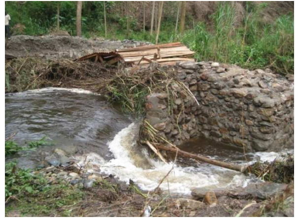
Fig 31.: Left: If there is a risk of heavy flooding, additional anchoring of the scaffold is required. Timber poles (A) stretching across from one abutment to the other will hold the scaffold together. They are the basis for additional poles which are nailed parallel with the abutments in the river bed. A large opening (B) should be left in the middle where the debris can pass. Right: The poles of the formwork in the middle caught the debris of the first seasonal floods. The water flow was blocked leading to serious damage and the river by-passing the structure.
