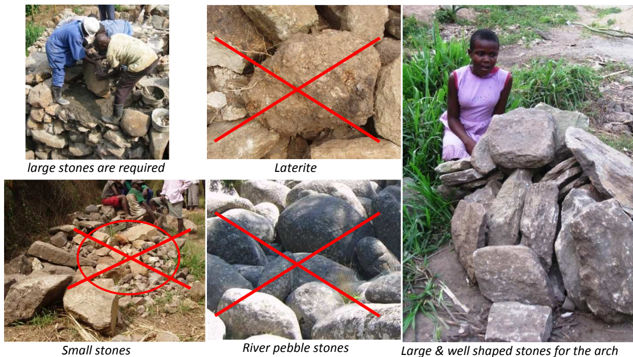
Fig. 44: Large stones make the bridge strong and reduce cost considerably. Prior to collection, the community should be given examples of the adequate stone size and the type of stones required.
