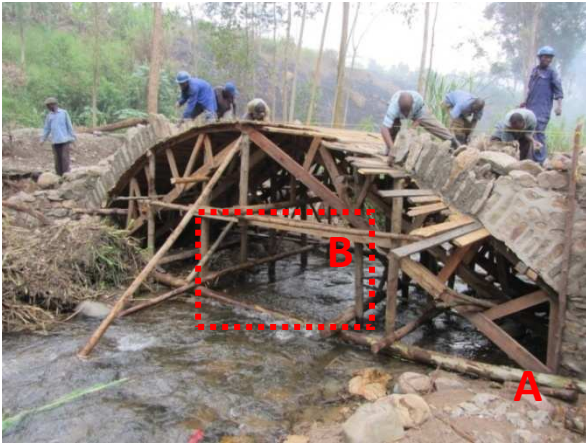
Fig 31.: Left: If there is a risk of heavy flooding, additional anchoring of the scaffold is required. Timber poles (A) stretching across from one abutment to the other will hold the scaffold together. They are the basis for additional poles which are nailed parallel with the abutments in the river bed. A large opening (B) should be left in the middle where the debris can pass. Right: The poles of the formwork in the middle caught the debris of the first seasonal floods. The water flow was blocked leading to serious damage and the river by-passing the structure.
