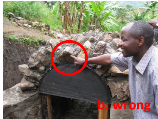
Fig. 40: a: Stones are tightly put together. They should act as a wedge with the narrow base pointing downwards. Fig 40 b: The keystone is wrongly placed. As the large base is at the bottom, the stone will fall out over time.
