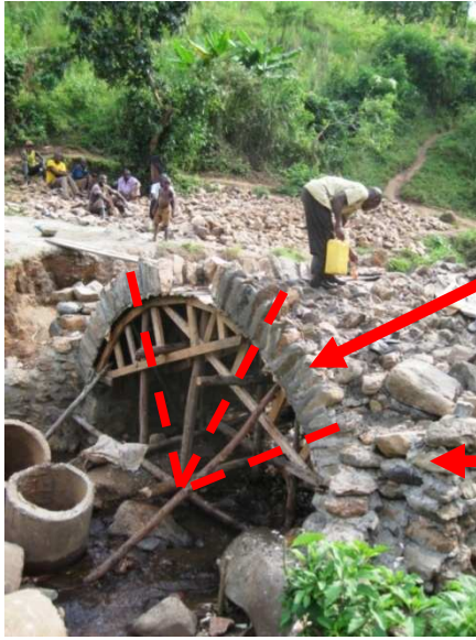
Fig. 24: Different positioning of stones in the structure
