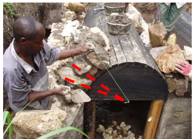
Fig. 37: Correct position of the stones along the radius of the arch. Stones of the arch are placed in a radial position, squared to the scaffold. A mason square indicates the correct position of each stone, provided the formwork is even. For culverts, a rope fixed in the centre of the circle can be used to show the right direction.
