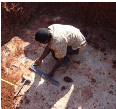
Setting out of foundations
