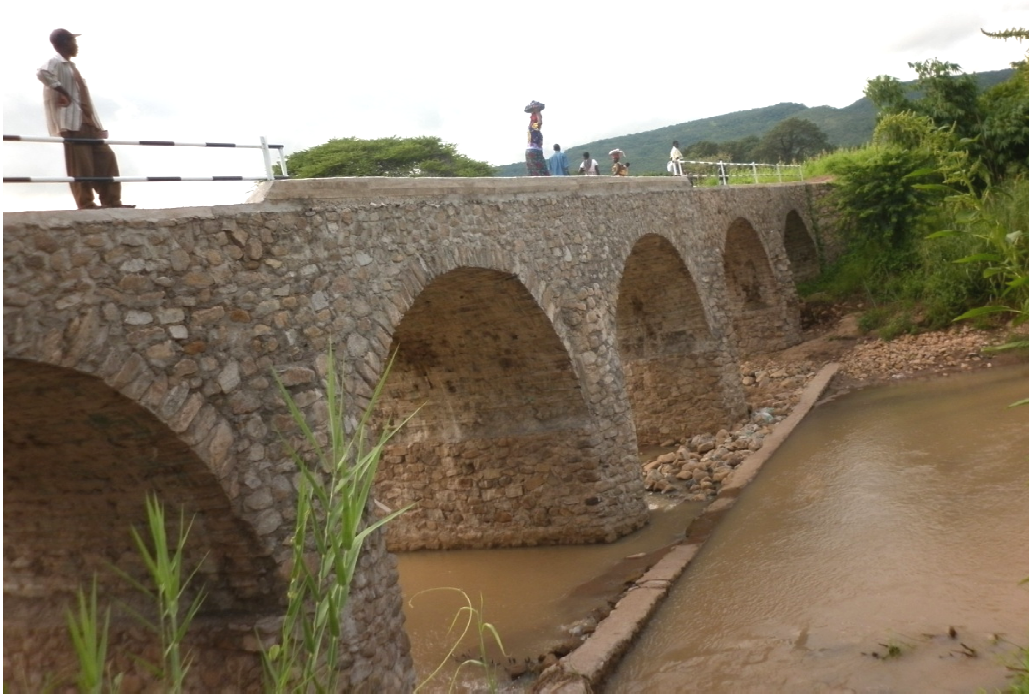
Fig 47: Multi stone arch bridges can be used to cover large spans. The span of this bridge was 50 metres and consisted of 5 arches. The picture is a courtesy of Rashid Mtamila/Tanzania.
