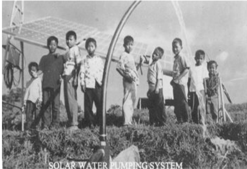
Solar Water Pump
