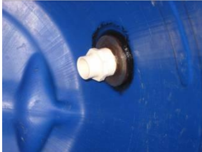
Inner hot water tank bulkhead fitting (inside the tank)
