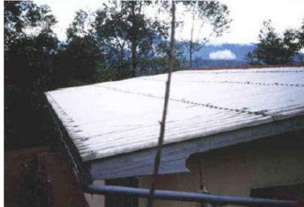
Figure 2: Typical Corrugated Iron Roof, Photo: Practical Action
