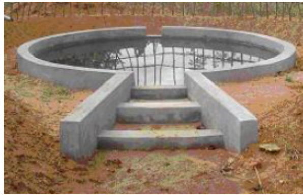
Figure 14: Runoff rainwater harvest tank Photo: Practical Action South Asia
