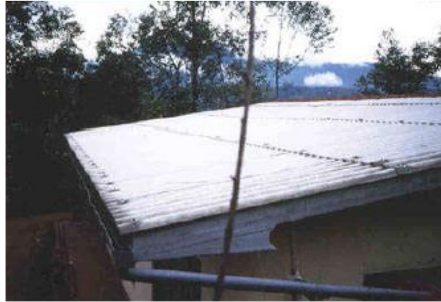
Figure 2: Typical Corrugated Iron Roof, Photo: Practical Action
