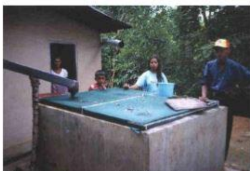
Figure 4a: An owner-built brick tank in Sri Lanka
