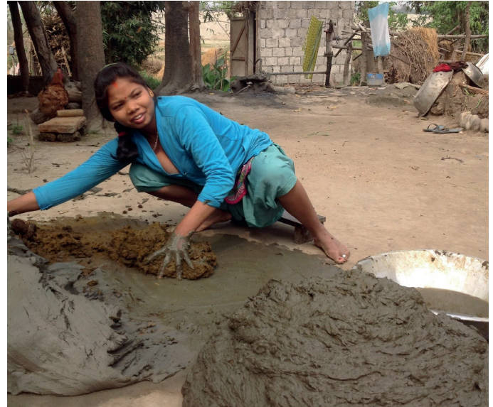
Figure 5: Woman in Rajapur arranging a mud dung paste for flooring in her house. Dung makes mud more resistant to disintegration and improves its capacity to absorb water. It also acts as a natural disinfectant and mosquito repellent, protecting residents from the spread of disease.
