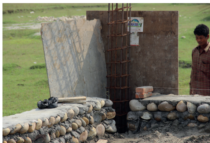
Figure 11: Building under construction. Note the ad-hoc, poorly constructed formwork and inadequate reinforcement. The local supply of materials was limited to smaller diameter, plain (non-deformed) bars with little attention to the use of steel links. Scrap timber boards are used to contain wet concrete, with little or no effective carpentry in evidence.
