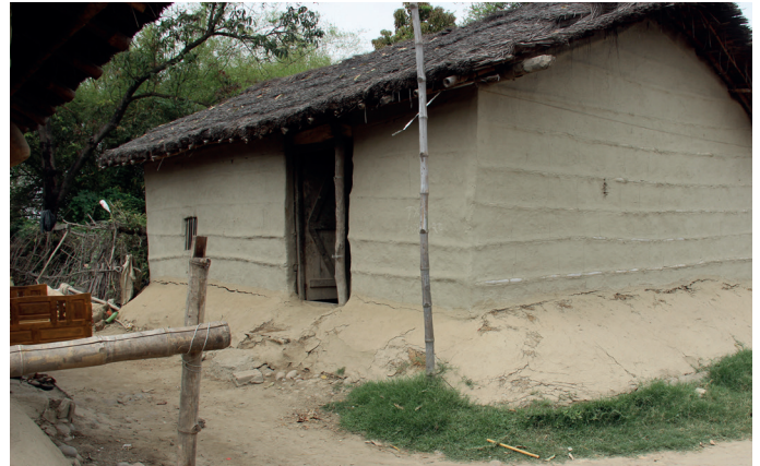
Figure 7: House with limited resilience, located less than 50 metres from the river. Constructed of timber, bamboo and earth, it sits on a slightly raised platform below the levels reached by water during flooding.
