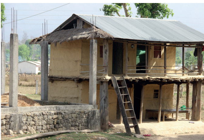
Figure 10: A new concrete house being built adjacent to a traditionally flood resilient house. Note the raised plinth platform and concrete pillars. Concrete represents a considerable financial investment compared to vernacular construction and may be perceived by local communities to be more resilient.
