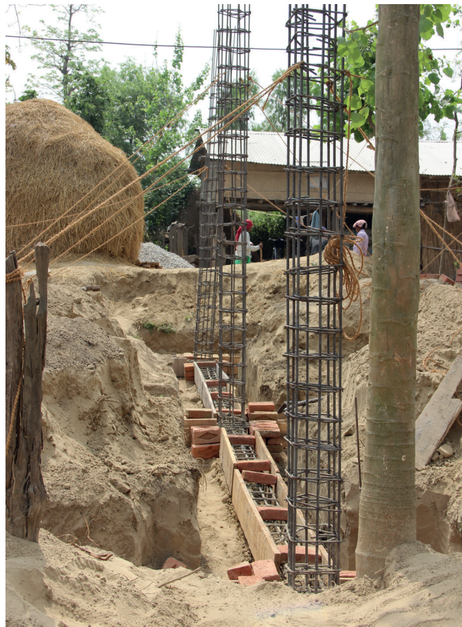
Figure 9: Engineered reinforcement for flood refuge shelters. Eight deformed steel bars, which have a rippled surface to attach more effectively to the concrete, are tied at frequent intervals with horizontal steel links for a robust structure. This type of reinforcement did not seem to be available at the local suppliers we visited.'
