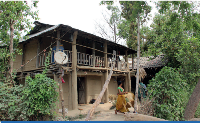
Figure 6: Traditionally constructed flood resilient house in Karnali. The main living space sits on a platform raised above the height of the highest flood level on moisture-resistant timber posts. The electrical supply to the house is connected just below roof level.
