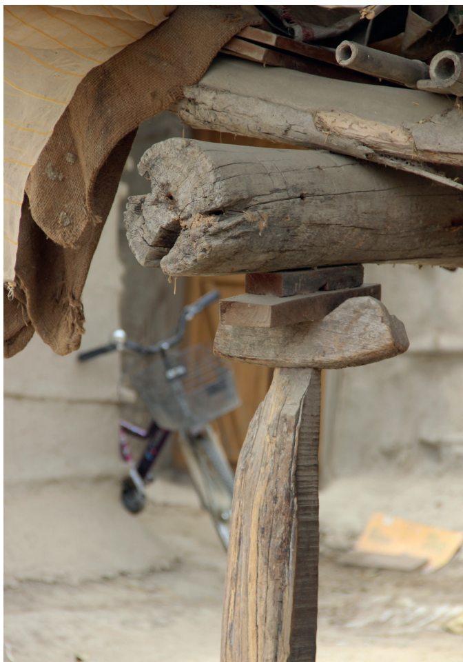
Figure 8: Ad-hoc timber construction. This image demonstrates a number of important points, the lack of availability or access to appropriate timber in long enough lengths, the use of random pieces of timber to provide additional height and little or no skill in carpentry to make an effective joint.
