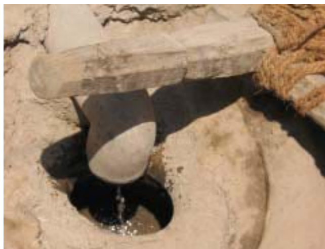
ABOVE AND LEFT A local community innovated this unique way of absorbing the wash-waste water from a wash room in to a perforated and buried earthen pot filled with pebbles and stones in a village in Maharashtra state in India. This kept the road dry and clean which used to be muddy and dirty before.
