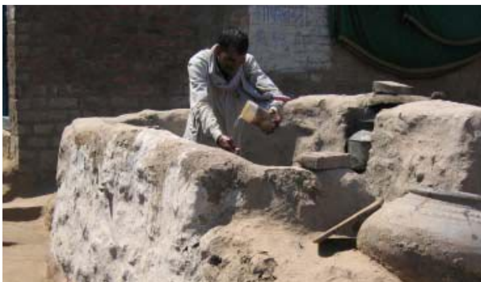
ABOVE Raised platform of a toilet to avoid seasonal flooding in Indonesia.
