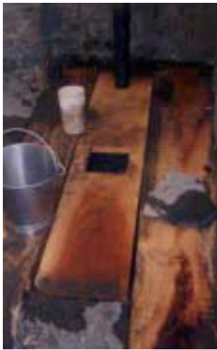
ABOVE Use of wooden planks in latrines built for the first time after triggering; Maharashtra, India.
