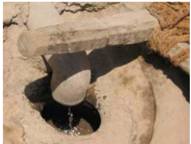
ABOVE AND LEFT A local community innovated this unique way of absorbing the wash-waste water from a wash room in to a perforated and buried earthen pot filled with pebbles and stones in a village in Maharashtra state in India. This kept the road dry and clean which used to be muddy and dirty before.
