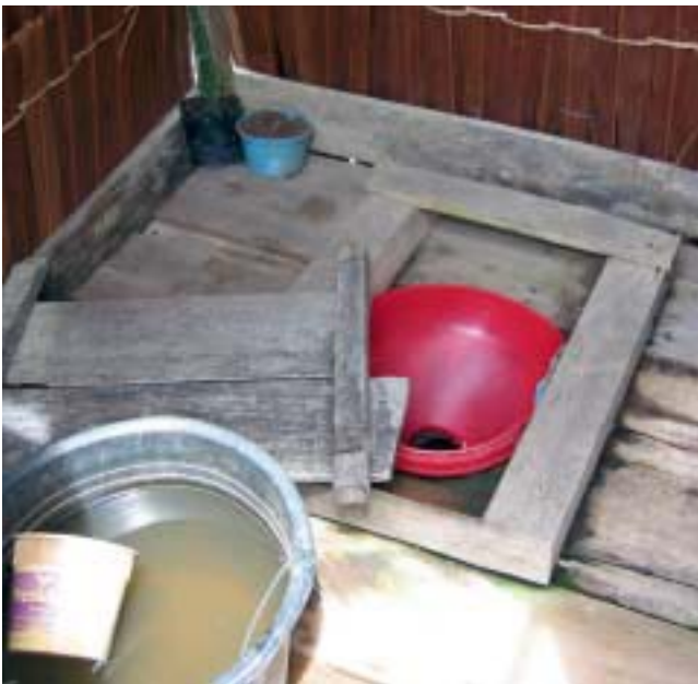
ABOVE A latrine constructed in South Sumatra, Indonesia. A woman used some household materials to construct a makeshift latrine in order to comply with the community's decision to go ODF, while her husband was away.
