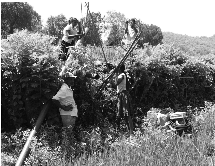
Figure 5: Women helping to lay the penstock at a pico hydro site
