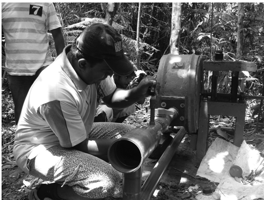
Figure 7: Assembling the turbine and penstock
