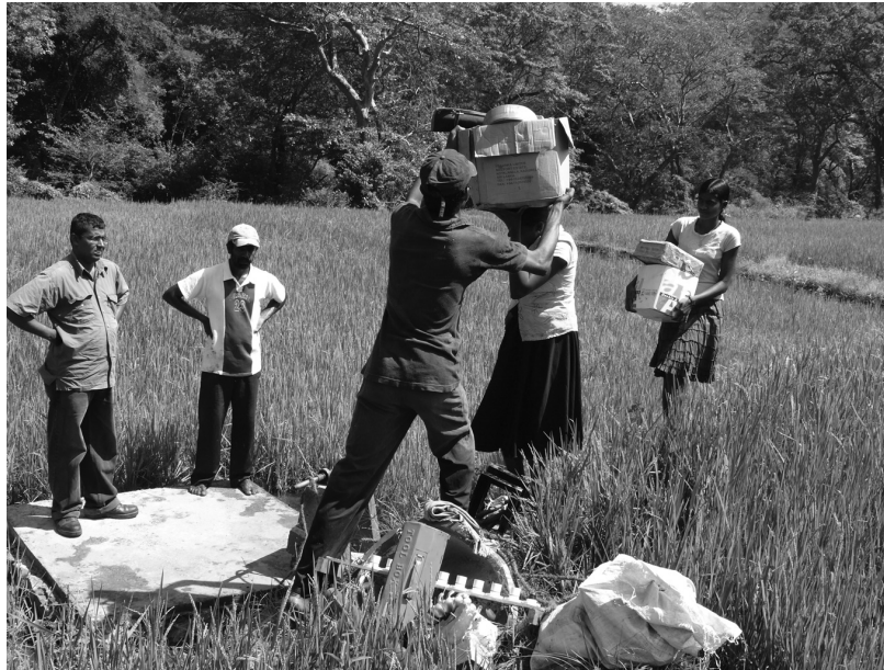
Figure 6: Women helping in the construction of a generator shed
