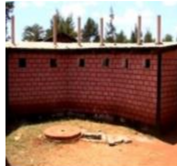
Figure 2: Large-scale biolatrone system showing the Biogas and toilet structures. Photo credit: Practical Action Kenya.
