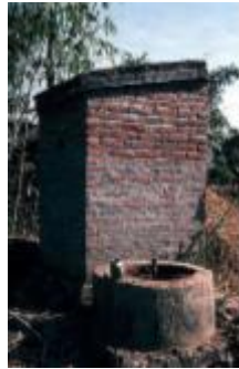
Figure 1: Household Biolatrone showing toilet attached to a bio-digester Photo credit: Practical Action. Nepal
