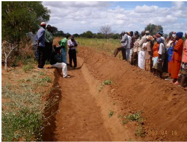
Figure 2: Complete dead level contour ready to harvest water. Photo: Practical Action, Southern Africa.
