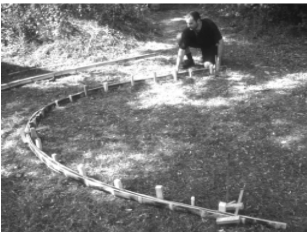
15-7 Construction of the arc with split bamboo
