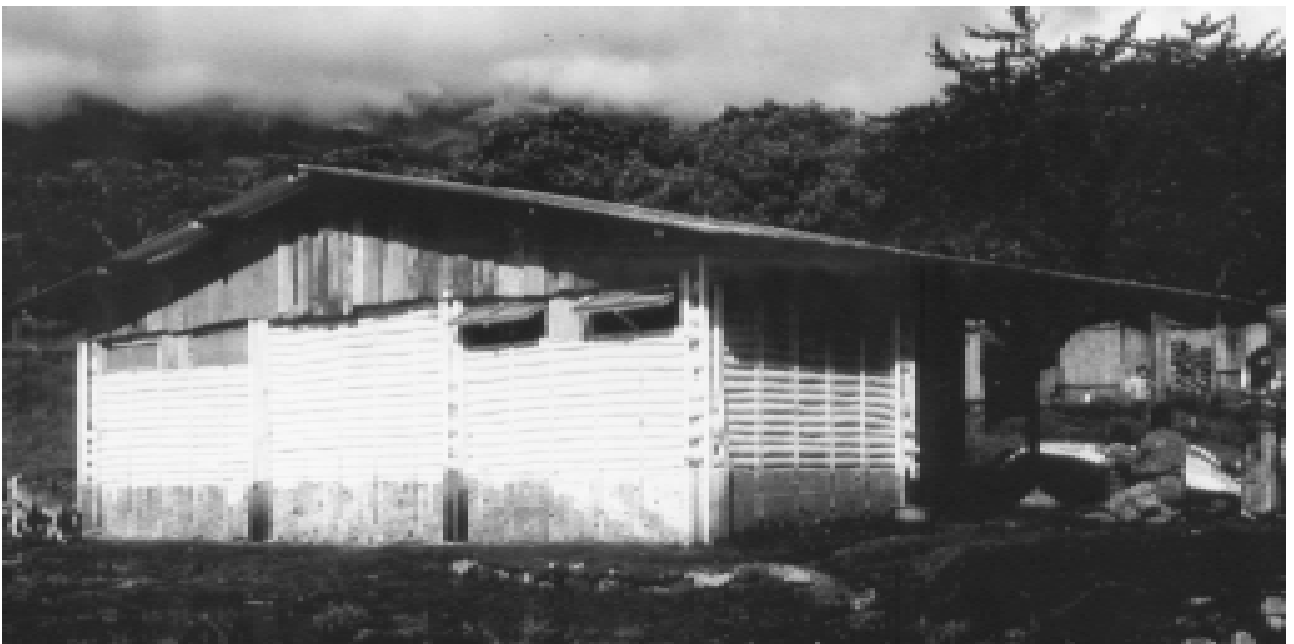
9-7 Earthquake resistant low-cost housing prototype, Guatemala 1978
