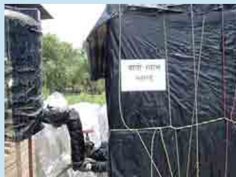
Biogas plant at WEPCO
