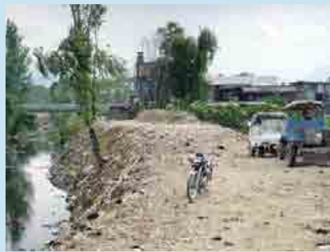
Filling with cover material (soil)
