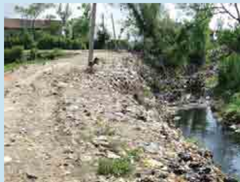
Road on old dumped waste
