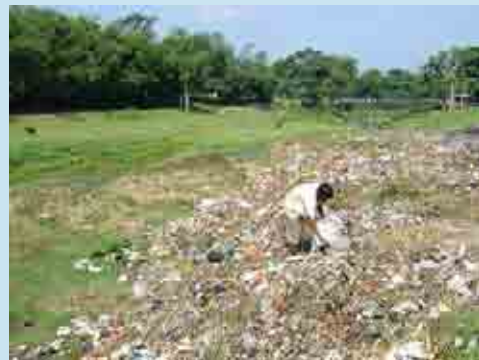
Covering the waste with ash to sanitise the dumping site
