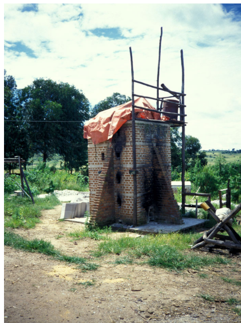
Figure 1: The construction of the experimental kiln, Dedza, Malawi. Photo credit: Practical Action/Kelvin Mason
