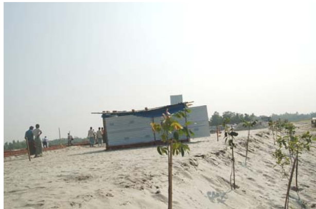
Figure 9: The newly finished earth raising is planted with young trees to stabilise the sandy soil. Photo: Practical Action Bangladesh.
