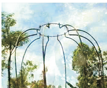
20- Tie ring to top of frames
