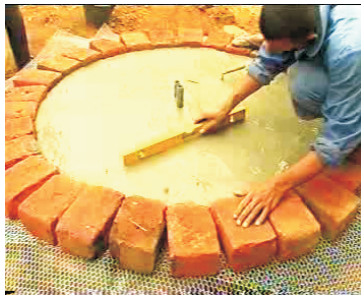
15- smoothen concrete surface
