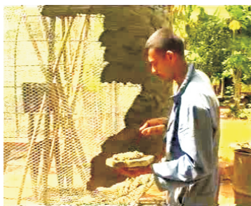
28- Place first layer of cement
