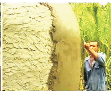
29- Place second layer of cement
