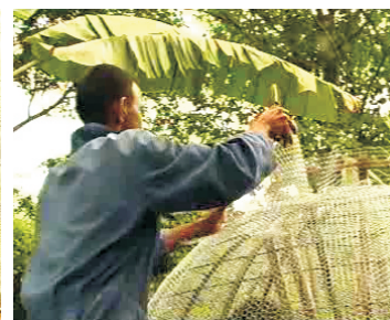
27- place mesh cylinder on tank
