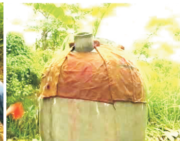
33- Allow tank to cure
