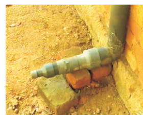
53- Fix stopper to runoff pipe
