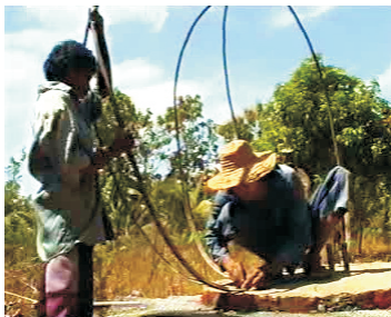
17- Fix the metal frames
