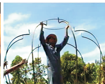
19- place ring at top of frames
