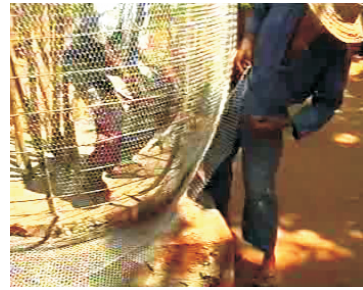
25- Fix base layers of mesh
