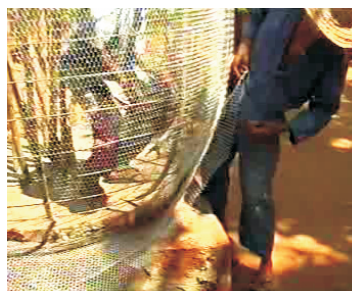
25- Fix base layers of mesh
