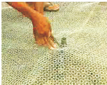
10- Cut mesh around pipes
