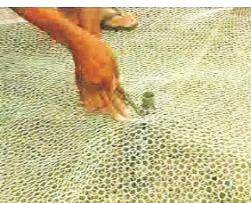
10- Cut mesh around pipes
