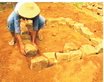
4- Cement the stone foundation
