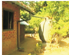
51- Install rain water pipes
