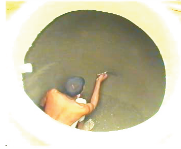
39- Smoothen inside with slurry
