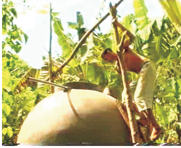
34- Erect scaffolding - enter tank
