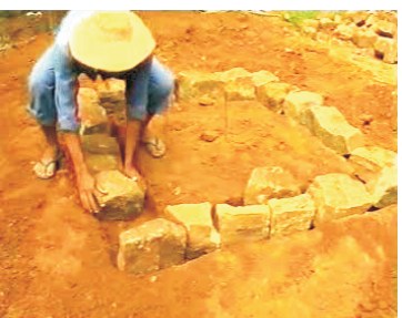
4- Cement the stone foundation
