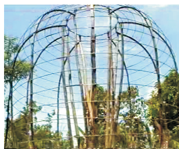
22- Place props inside framework
