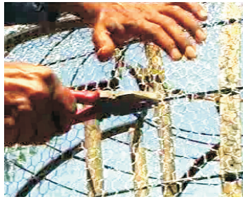
24- Fix chicken mesh to frames
