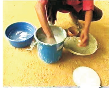
38- Prepare waterproof slurry
