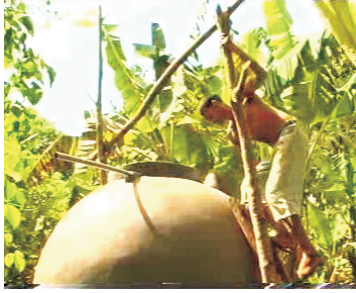
34- Erect scaffolding - enter tank
