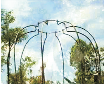
20- Tie ring to top of frames
