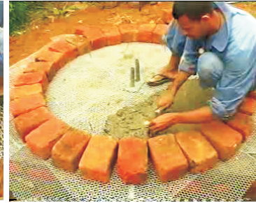
14- Lay concrete within brick circle
