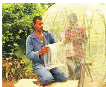
26- Fabricate mesh cylinder
