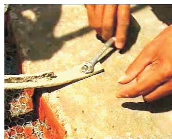
18- Tighten nuts at frames
