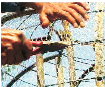
24- Fix chicken mesh to frames
