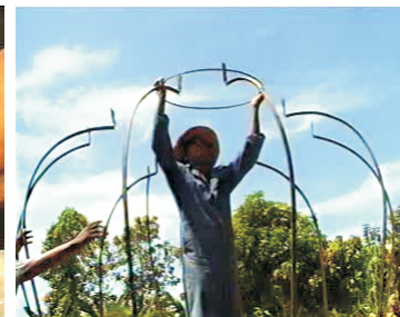
19- place ring at top of frames
