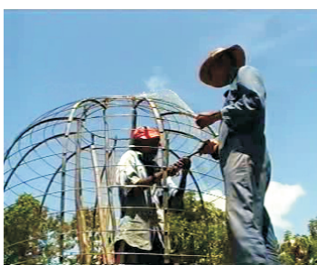
21- Fix metal hoops to frames
