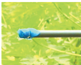
50- Tie net on overflow pipe
