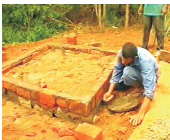
5- Cement the brick layer
