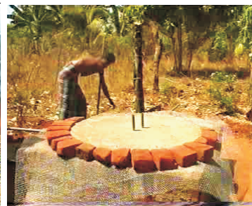
16- Remove row of bricks
