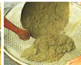
42- Lay cement on mesh
