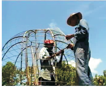
21- Fix metal hoops to frames
