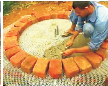
14- Lay concrete within brick circle
