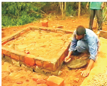
5- Cement the brick layer
