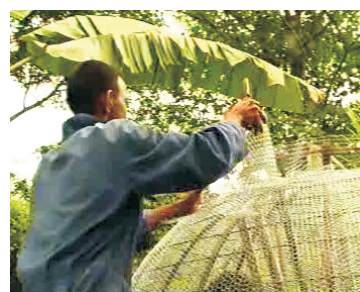
27- place mesh cylinder on tank
