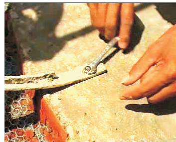
18- Tighten nuts at frames
