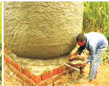
30- Place cement at base
