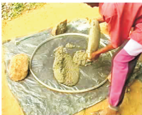
40- Place cement in MS ring
