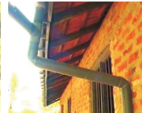
52- Install run-off pipe
