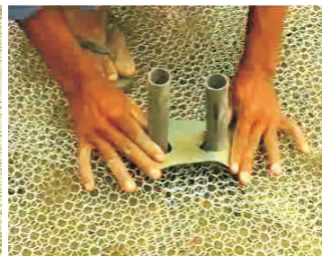
11- Place PVC strip at pipes
