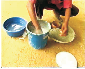
38- Prepare waterproof slurry
