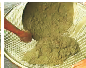
42- Lay cement on mesh
