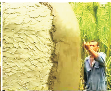
29- Place second layer of cement
