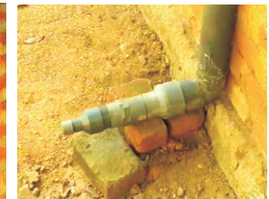
53- Fix stopper to runoff pipe
