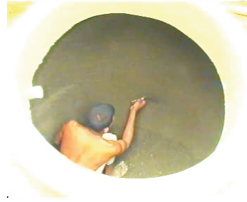
39- Smoothen inside with slurry
