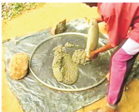
40- Place cement in MS ring
