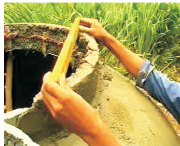
32- Smoothen lip of tank
