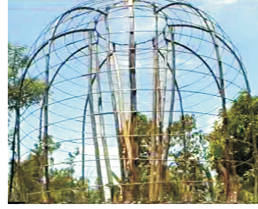
22- Place props inside framework
