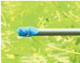
50- Tie net on overflow pipe
