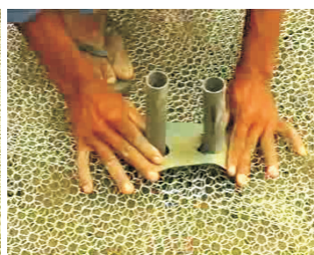
11- Place PVC strip at pipes
