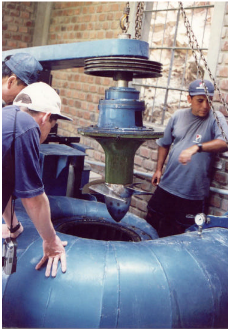
Fig. 6 Joining of the shaft and components to the frame.
