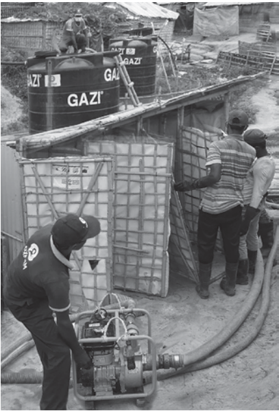
Figure 7.4 Pit emptying using centrifugal pump
