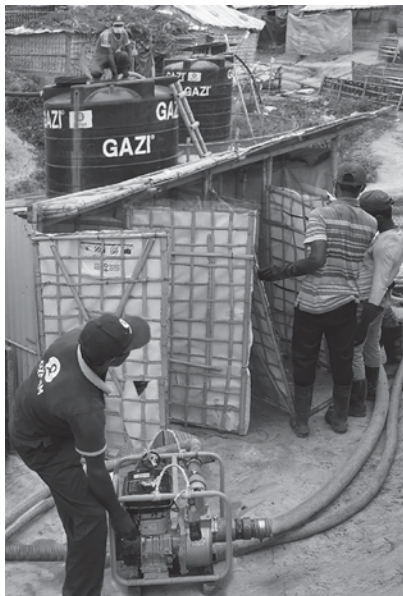
Figure 7.4 Pit emptying using centrifugal pump
