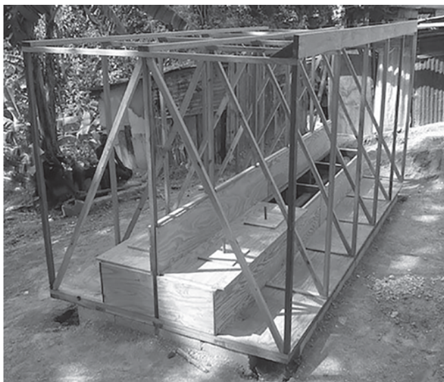
Figure 6.9 Construction of a pedestal trench toilet
