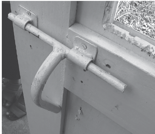
Figure 5.6 Large door bolt, easy to grasp Note: The small window allows the door to be opened from the outside in an emergency. Source: (** Jones & Reed, 2005)
