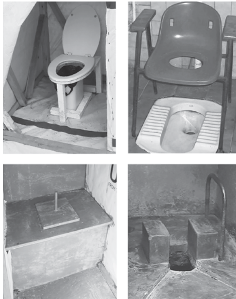
Figure 5.12 Dry pedestal interfaces
