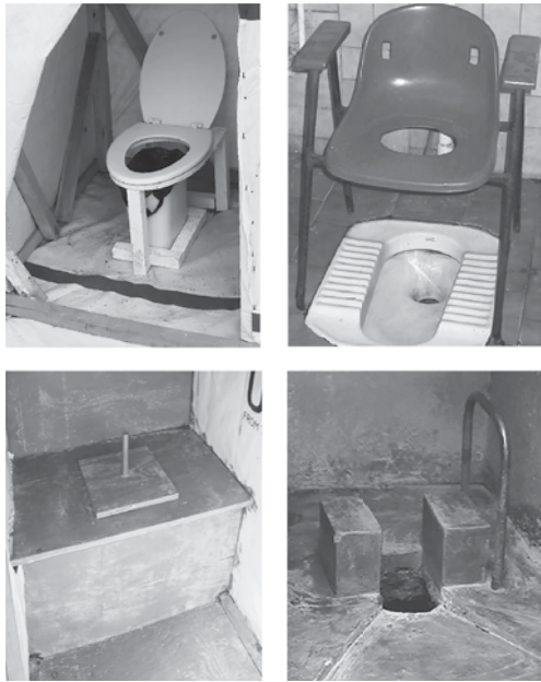
Figure 5.12 Dry pedestal interfaces
