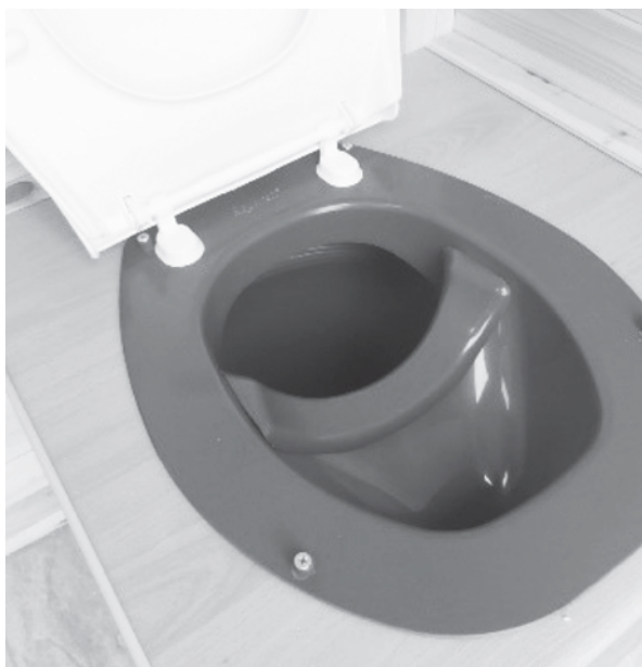
Figure 5.13 Urine diversion interface
