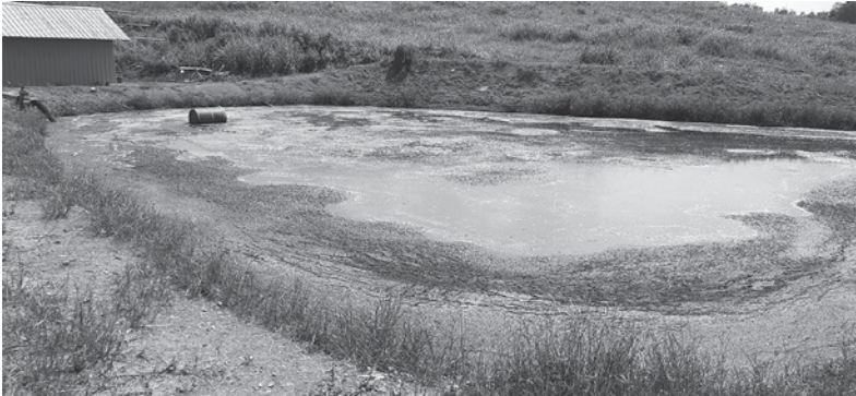
Figure 9.9 Anaerobic waste stabilization pond
