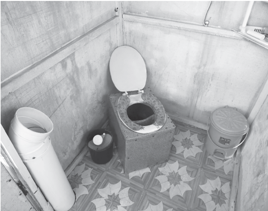
Figure 11.4 Toilet cubicle in a cold region
