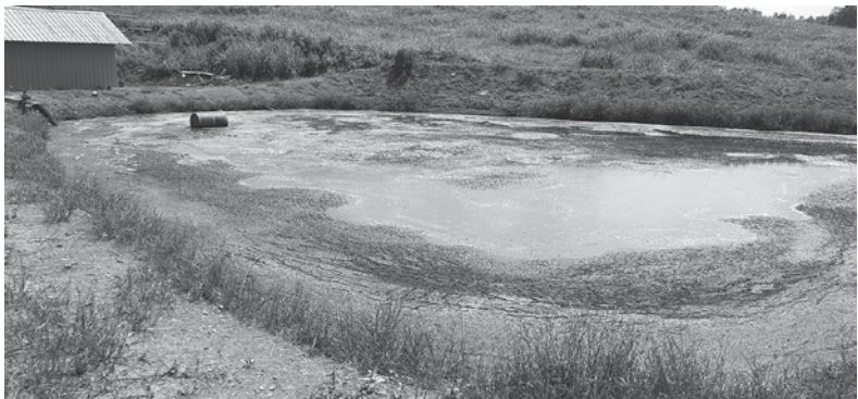
Figure 9.9 Anaerobic waste stabilization pond
