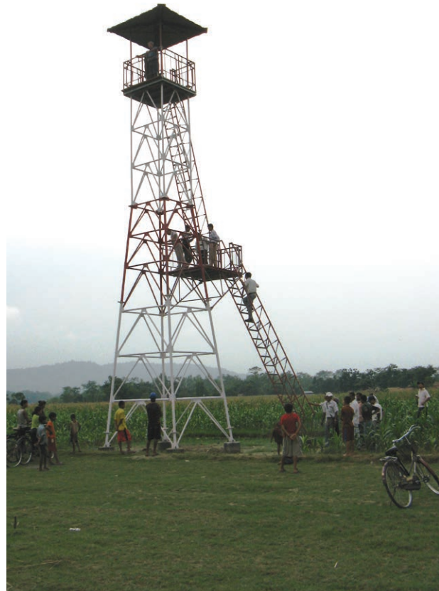
Photo 4: Modified EWS tower in Meghauli, Chitwan
