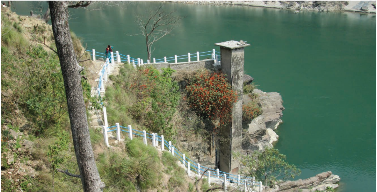
Photo 7: River gauge station at Chisapani, Karnali River
