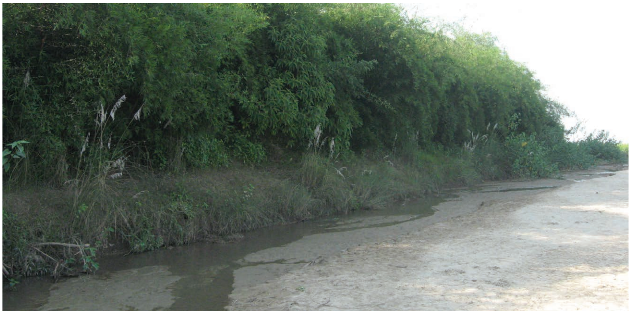
Photo 6: Bio-dyke along the river to reduce the bank cutting
