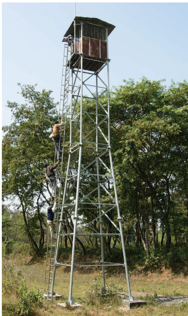
Photo 1: The first EWS tower in Bhandara, Chitwan
