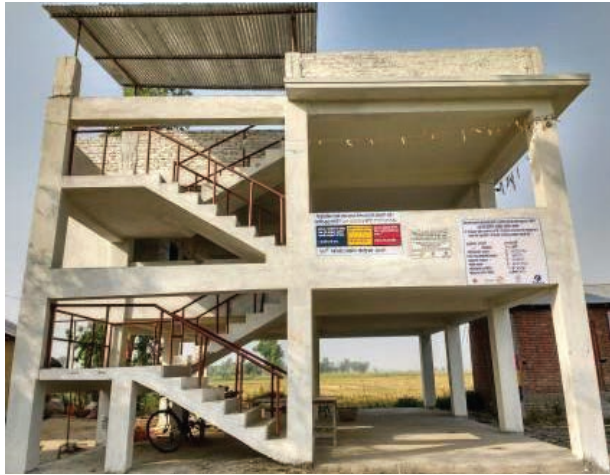
Photo 10: Flood emergency shelter
