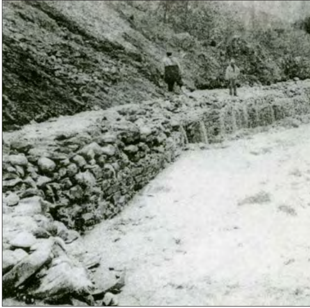
Photo 3.11 Gabion walls at the headworks of the 30kw Jharkot micro-hydro scheme, Mustang, Nepal.
