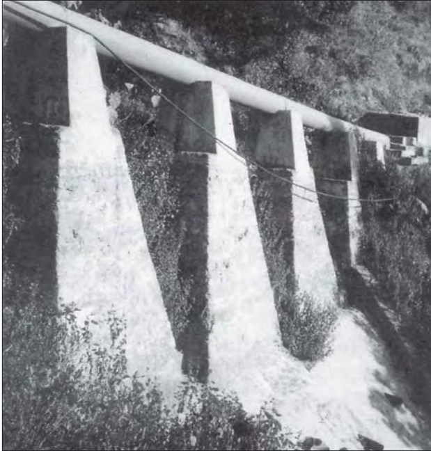
Photo 4.14 Jhankre mini-hydro penstock crossing, Dolakha, Nepal.
