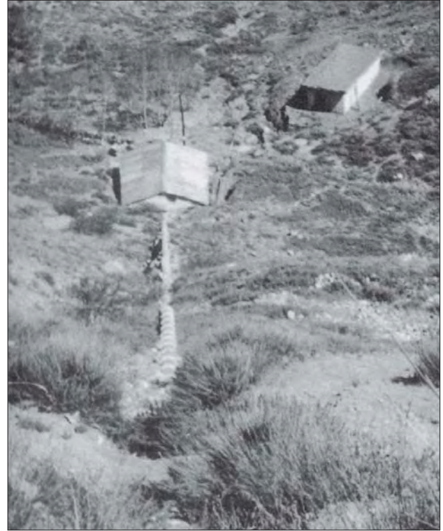
Photo 6.1 Penstock alignment of the 36 kW Jharkot micro-hydro scheme, Mustang, Nepal
