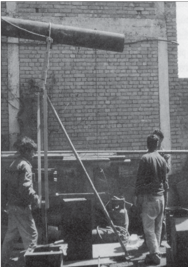
Photo 10.7 Load test of steel support pier (side elevation)
