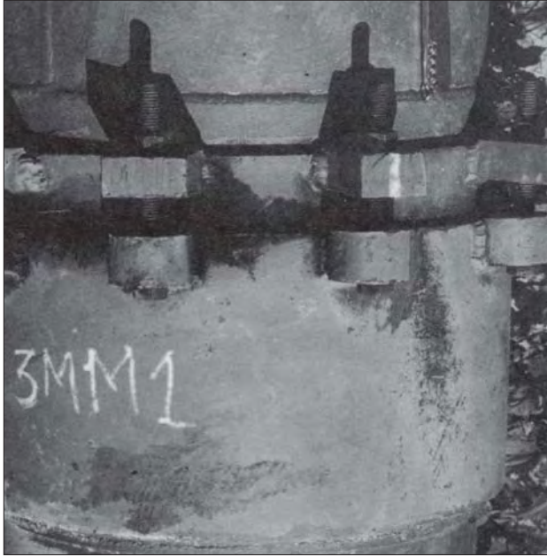
Photo 6.13 Sliding expansion joint, Jhankre mini-hydro
