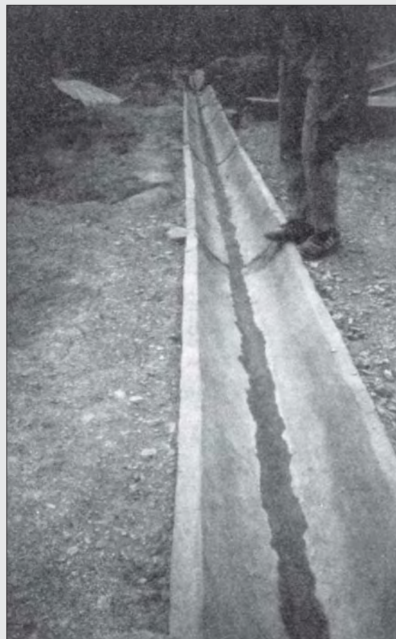
Photo 4.8 Andhi Khola Project ferrocement flume
