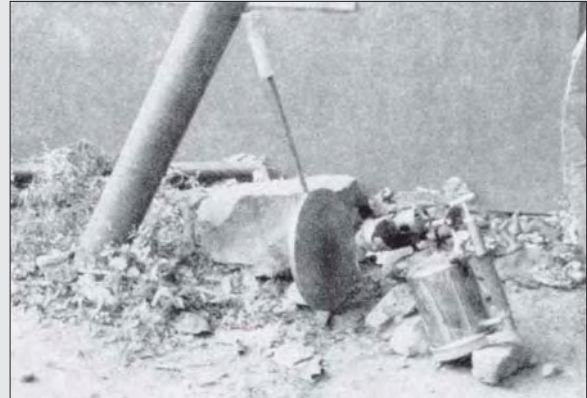
Photo 4.20 Heating the welding plate
