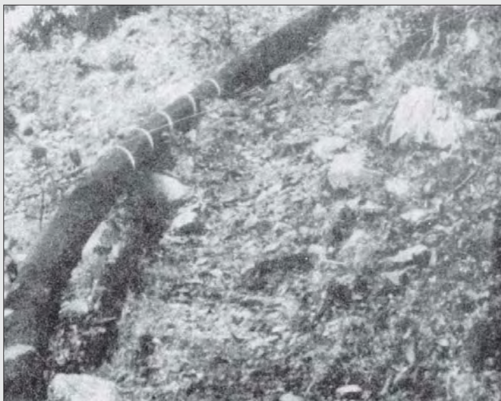
Photo 4.18 HDPE headrace pipe along unstable alignment, Ghandruk micro-hydro scheme, Nepal.
