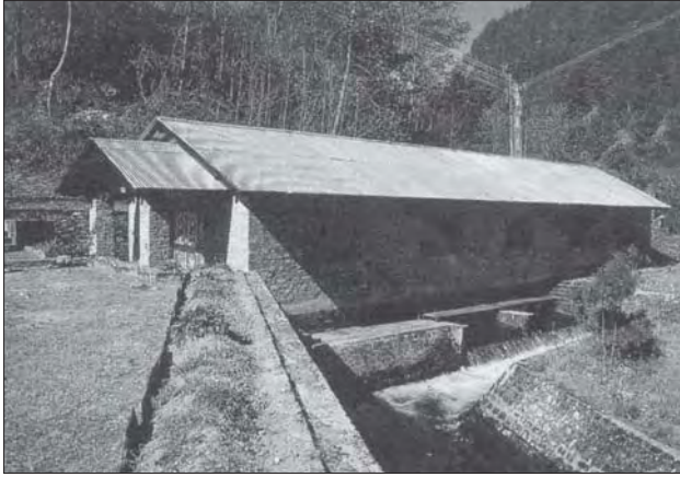
Photo 8.2 Powerhouse and tailrace of the Salleri Chialsa mini-hydro scheme
