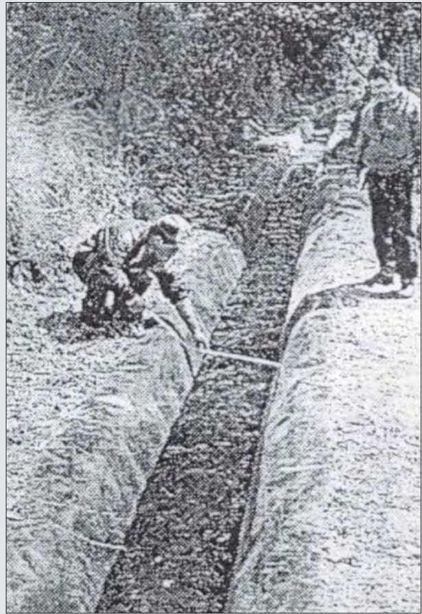
Photo 4.9 HDPE lining at El Tinte, Peru
