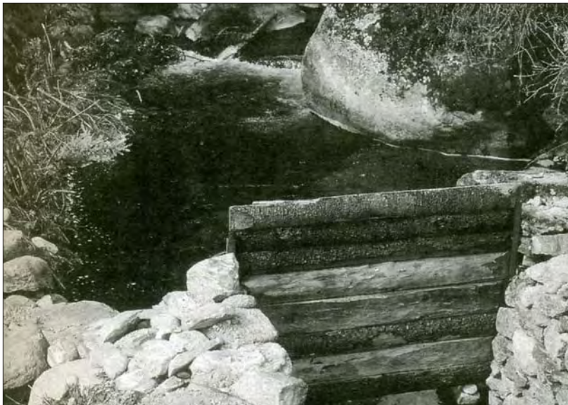
Photo 3.5 Timber planks placed horizontally in grooves provide a low-cost gate in a channel. In this case, the timbers have been lifted to act as a restricting orifice (Mhapung)
