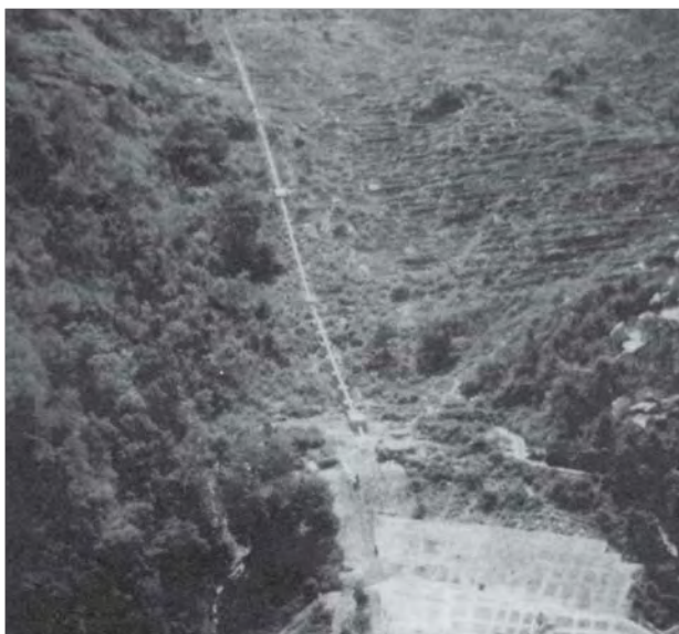
Photo 6.9 Jhankre mini-hydro penstock alignment
