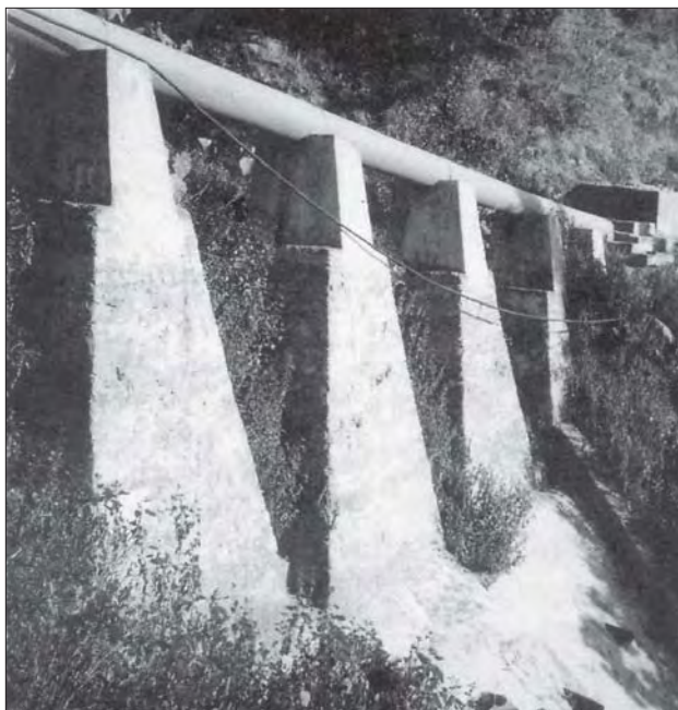
Photo 4.14 Jhankre mini-hydro penstock crossing, Dolakha, Nepal.
