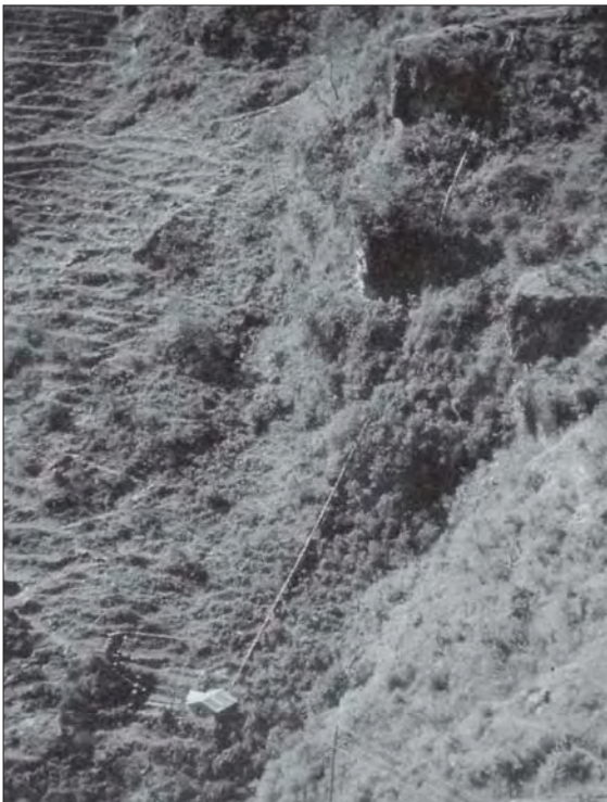
Photo 6.2 Penstock alignment of the 50 KW Barpak micro-hydro scheme, Gorkha, Nepal
