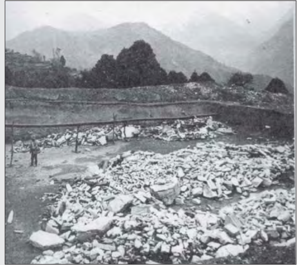
Photo 5.14 Ghandruk peaking reservoir during construction
