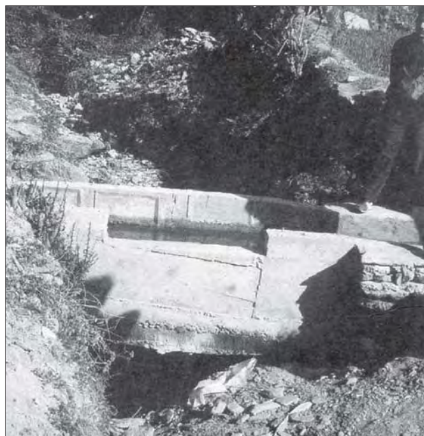
Photo 4.12 Spillway on a crossing where the excess flow is discharged into a gully, Galkot micro-hydro scheme, Baglung, Nepal.
