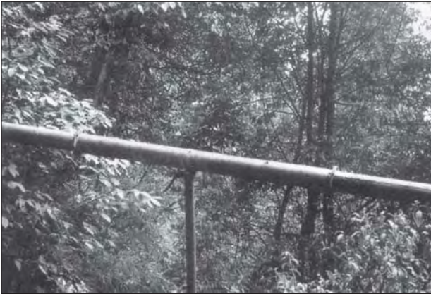
Photo 4.15 Jhankre mini-hydro headrace crossing Ghandruk, Nepal.
