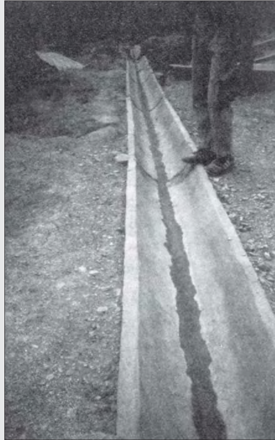
Photo 4.8 Andhi Khola Project ferrocement flume
