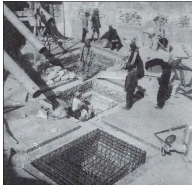
Photo 8.4 Construction of Jhankre mini-hydro machine foundation.
