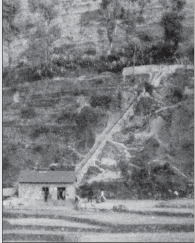
Photo 6.8 Penstock alignment, Galkot
