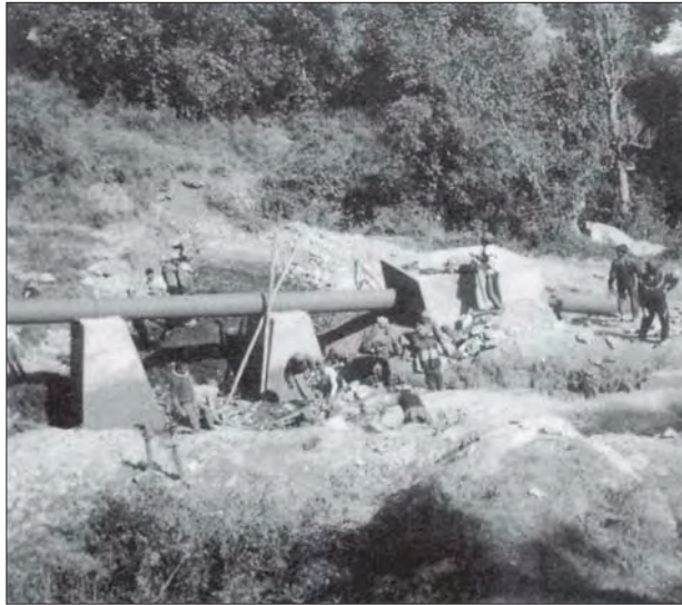
Photo 7.5 Stone masonry support piers, Jhankre mini-hydro scheme
