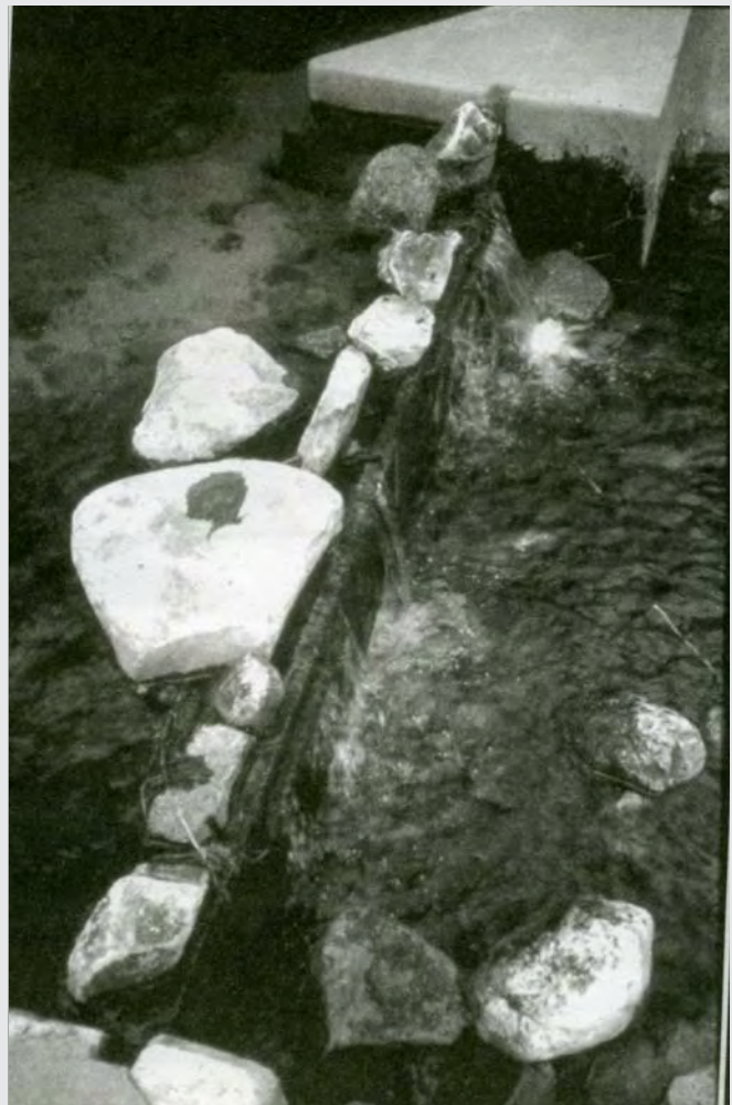
Photo 3.8 Slotted concrete piers
