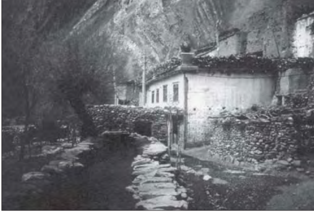
Photo 4.2 A raised masonry channel supplying a mill (Mustang).
