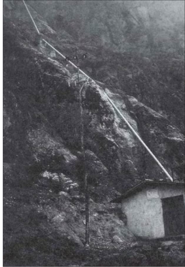
Photo 6.4 penstock installation is often challenging and requires safe and careful work.
