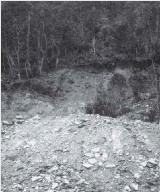
Photo 9.5 Excavated slope at powerhouse
