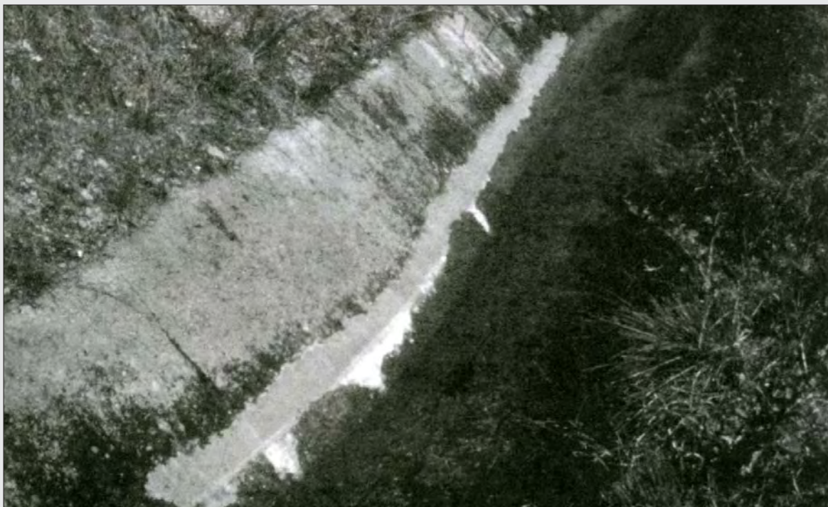
Photo 4.10 Soil cement lined canal section at Andhi Khola , Nepal.
