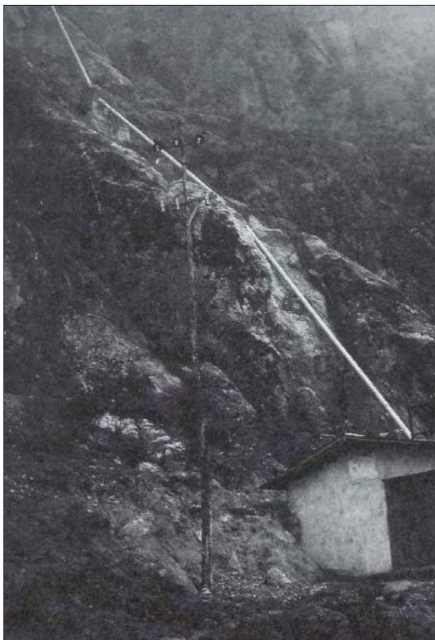
Photo 6.4 penstock installation is often challenging and requires safe and careful work.
