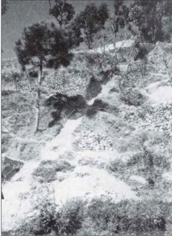
Photo 6.7 Excavation for penstock alignment, Galkot
