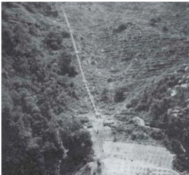
Photo 6.9 Jhankre mini-hydro penstock alignment
