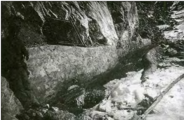
Photo 3.10 Bottom intake with the grill removed (Jhong)
