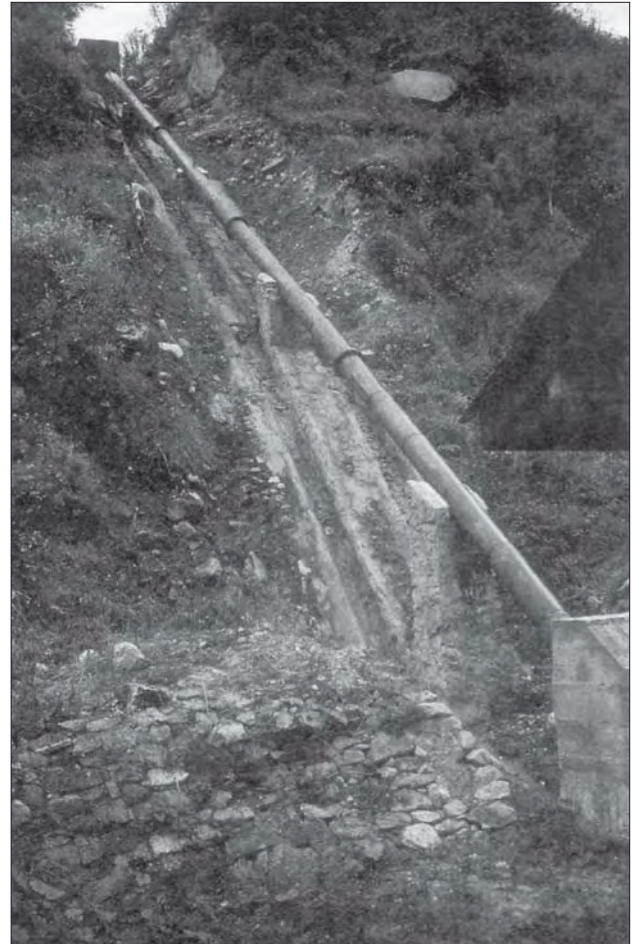
Photo 7.1 A straight penstock with four supports and an anchor block before the power house
