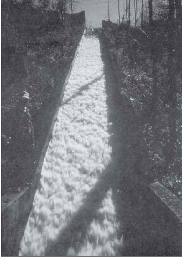
Photo 8.6 Tailrace channel of the Jhankre mini-hydro scheme
