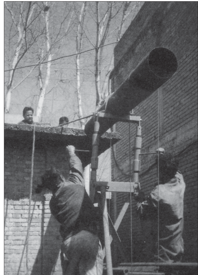
Photo 10.8 Load test of steel support pier (front elevation)
