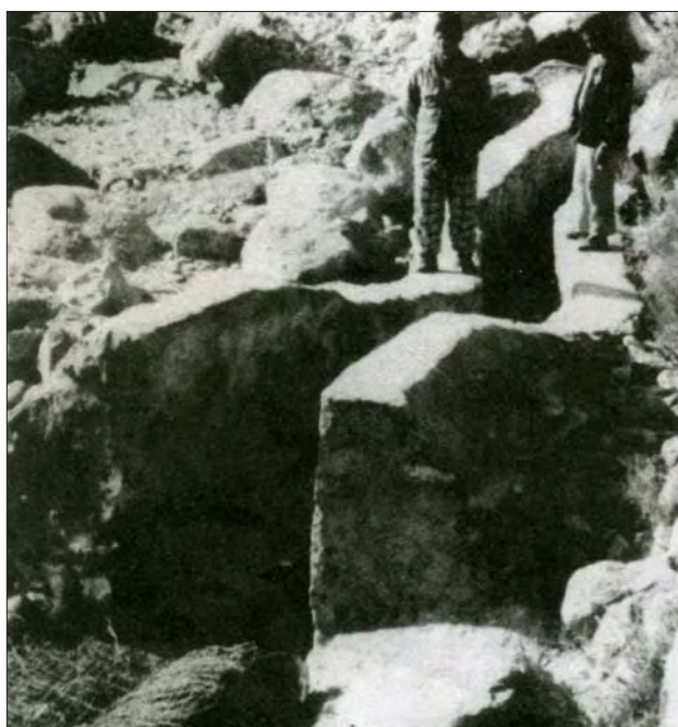
Photo 3.2 Side intake of the Galkot micro-hydro scheme, Baglung, Nepal (see Appendix C for drawing)
