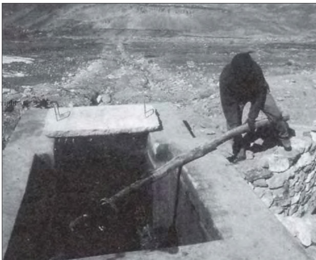
Photo 5.3 Lifting the flushing mechanism (Jhong)
