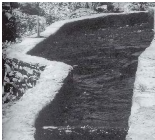
Photo 5.1 Galkot gravel trap
