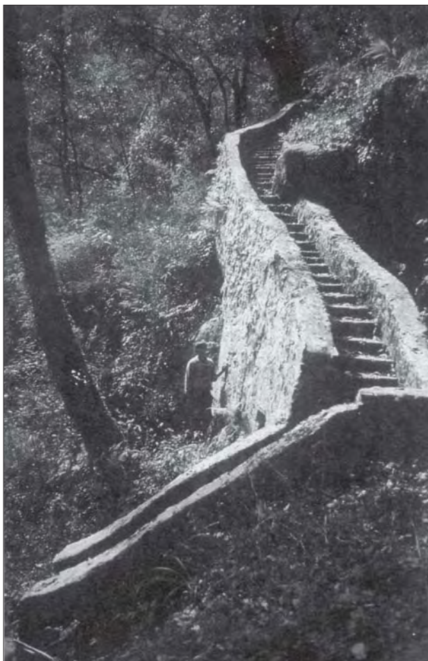
Photo 9.2 Masonry steps for energy dissipation and control of spillway water. Although costly, elaborate control is essential where slopes are vulnerable to erosion (Siklis)
