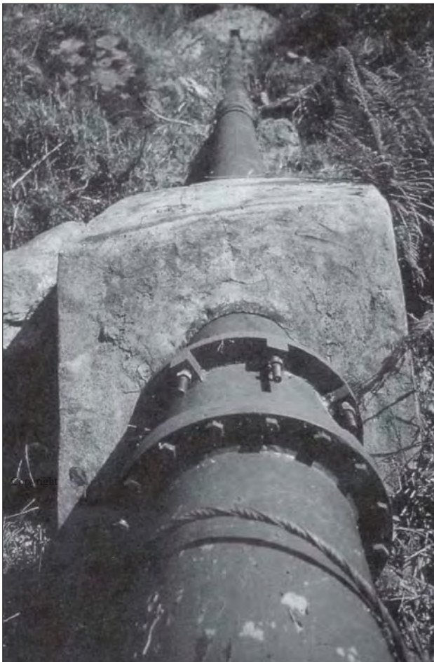
Photo 6.12 An expansion joint should be located just below an anchor block to protect the block from forces which it may not be designed to resist (Siklis)
