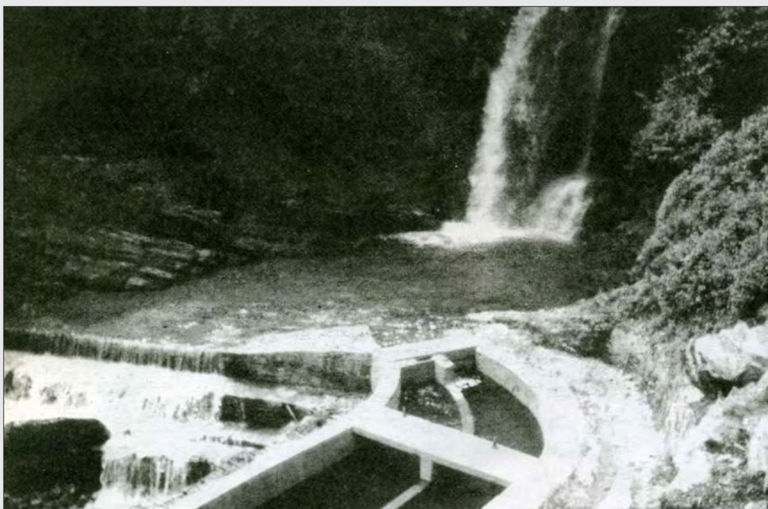
Photo 3.7 Diversion weir of the Jhankre Mini-Hydro Scheme
