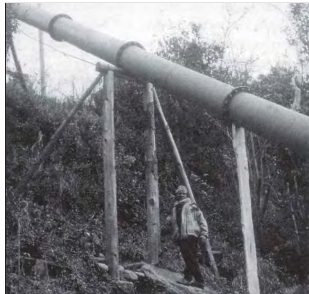
Photo 7.7 Wooden support piers at Kamche micro-hydro, Nepal
