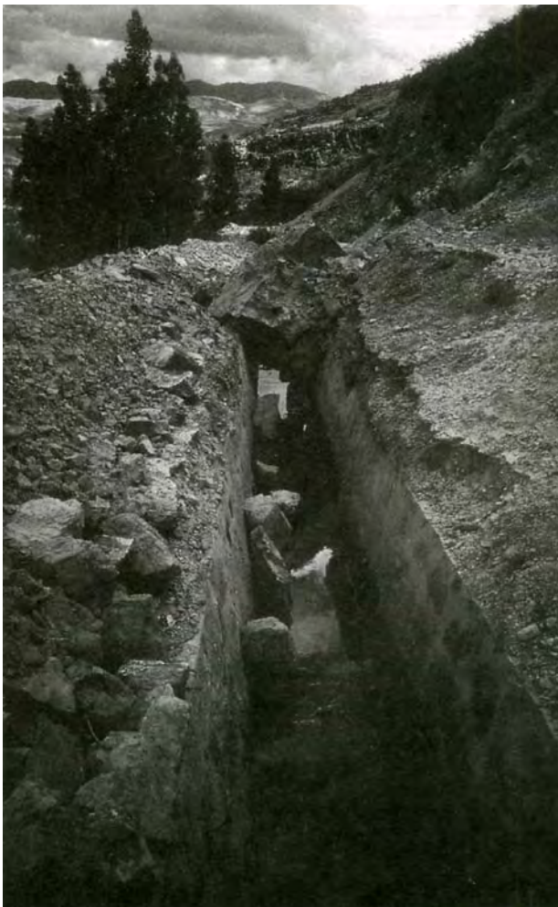
Photo 2.2 Obstruction caused by debris falling from on unstable slope
