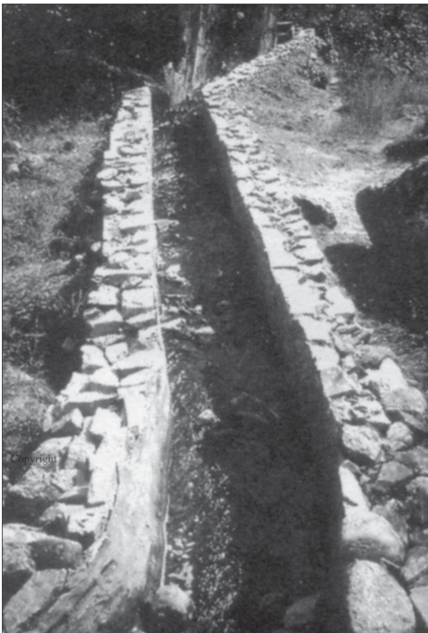
Photo 4.3 Stone masonry in cement mortar headrace canal of the 50kw Galkot MHP, Galkot, Baglung, Nepal.
