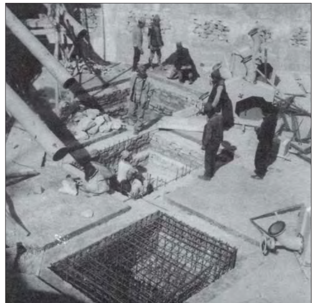
Photo 8.4 Construction of Jhankre mini-hydro machine foundation.
