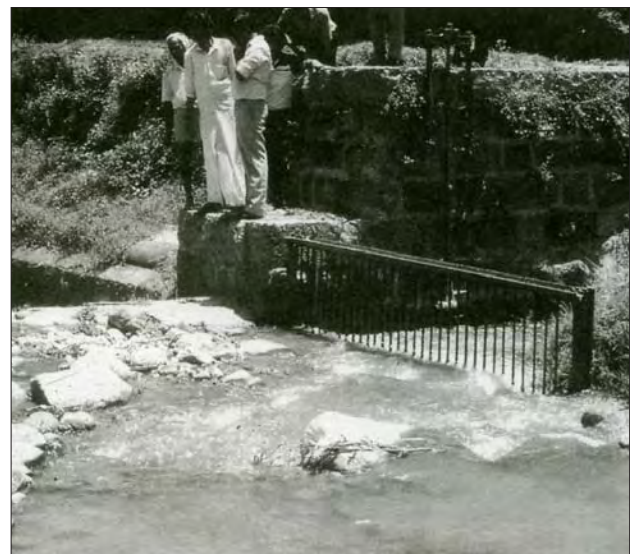
Photo 3.3 Where an intake is liable to attract floating debris a trashrack may be necessary ( Sri Lanka )
