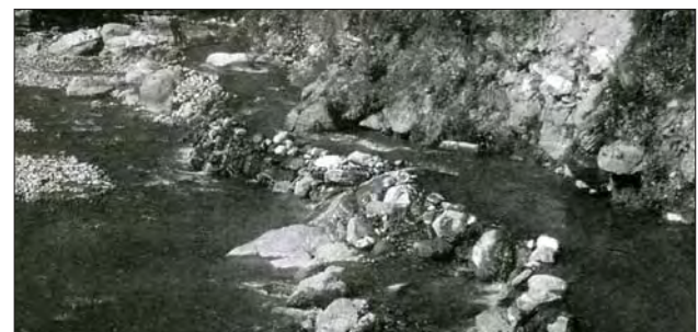
Photo 3.6 A temporary weir in Type 2B river (Dhading)
