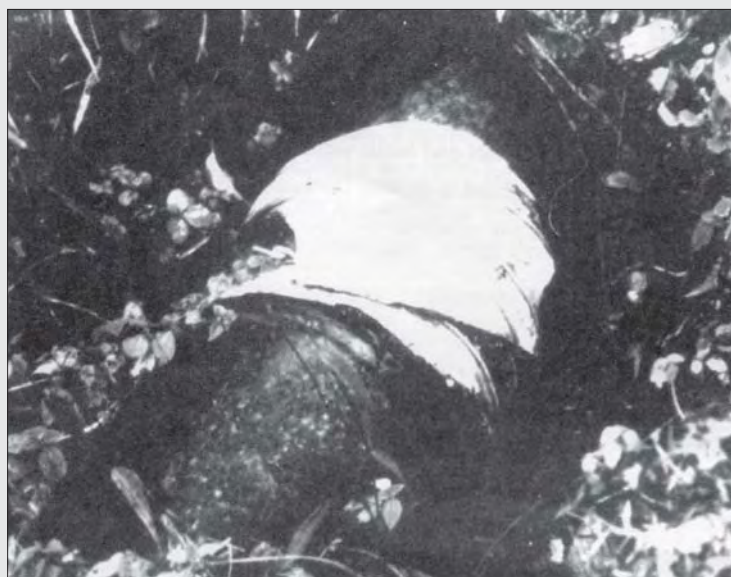
Photo 4.19 Bend prepared by cutting and welding the HDPE headrace pipe at Ghandruk
