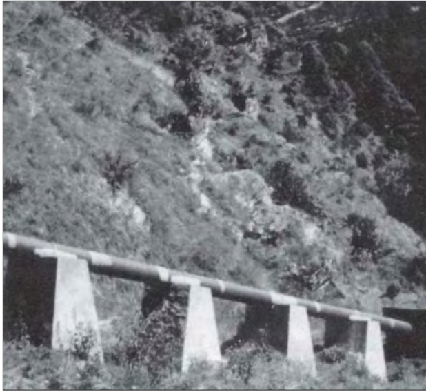
Photo 6.5 Penstock alignment high above the ground to allow access for people and cattle, Jhankre mini-hydro
