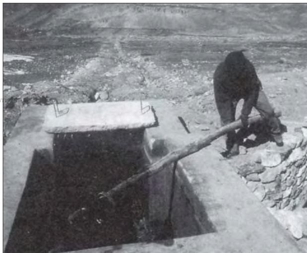
Photo 5.3 Lifting the flushing mechanism (Jhong)
