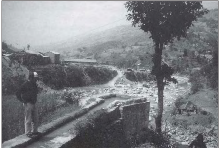
Photo 5.10 A cement masonry channel and forebay at the top of a steep slope (Dhading)
