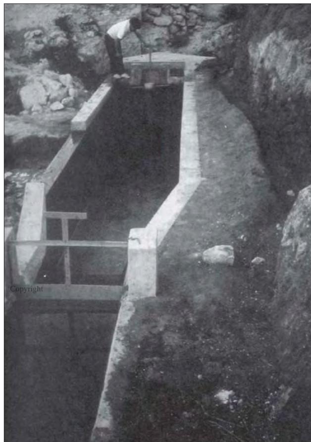
Photo 5.2 Sliding gate at settling basin entrance, Peru
