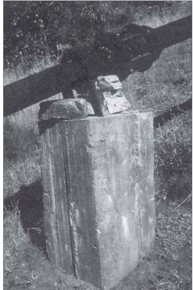
Photo 7.6 The use of an extension to the concrete support lifts the pipe clear of an pier, allowing drainage and preventing corrosion between the pier and the pipe (Khamche)
