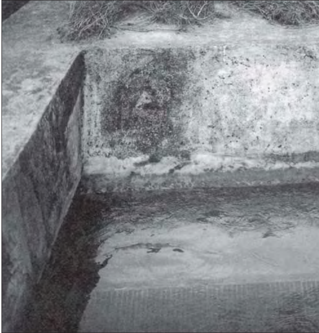
Photo 5.12 Submerged trashrack, Salleri Chialsa mini-hydro scheme
