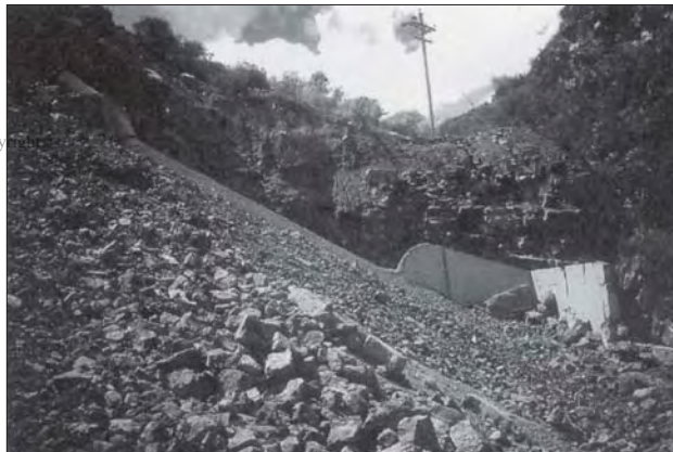
Photo 9.1 Unstable slopes are a threat to schemes. This powerhouse was destroyed by a landslide
