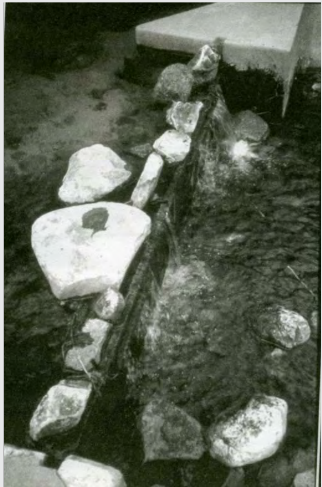
Photo 3.8 Slotted concrete piers
