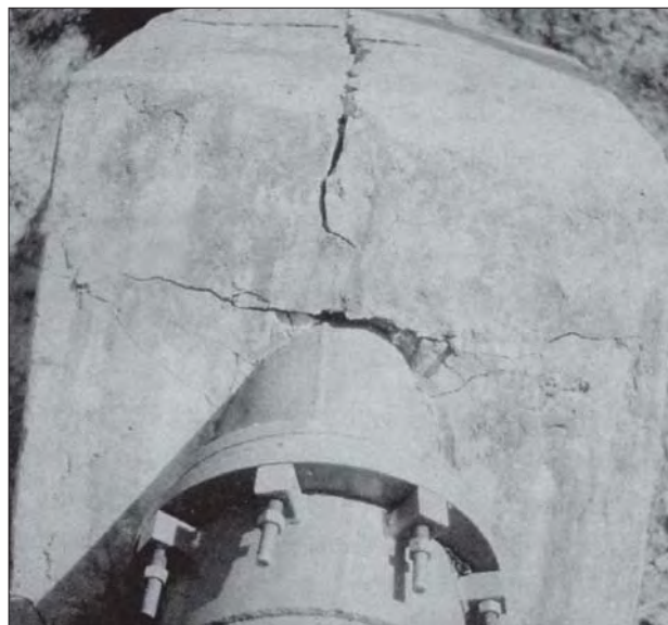
Photo 7.3 Cracking of the upper surface of an unreinforced anchor block
