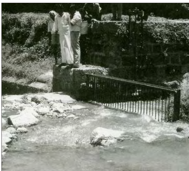
Photo 3.3 Where an intake is liable to attract floating debris a trashrack may be necessary (Sri Lanka)
