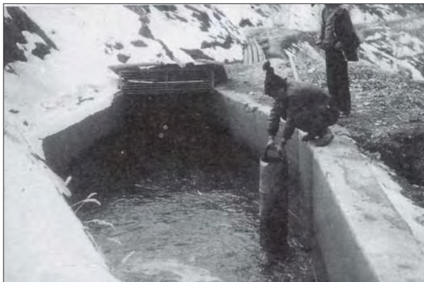
Photo 5.5 Settling basin at Jharkot
