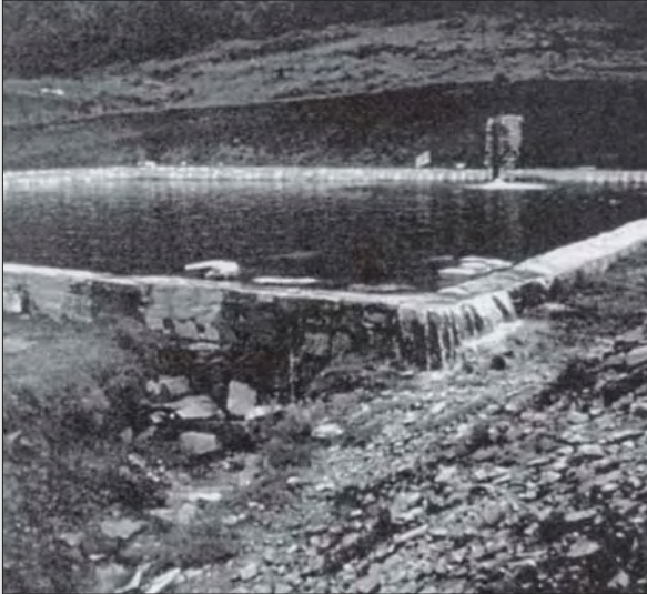
Photo 5.15 Ghandruk peaking reservoir after construction
