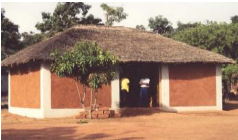
Figure 4: Demonstration house in Jos, Nigeria, built with adobe laid in mud mortar and plastered with mud mortar. Photo: CRATerre/EAG
