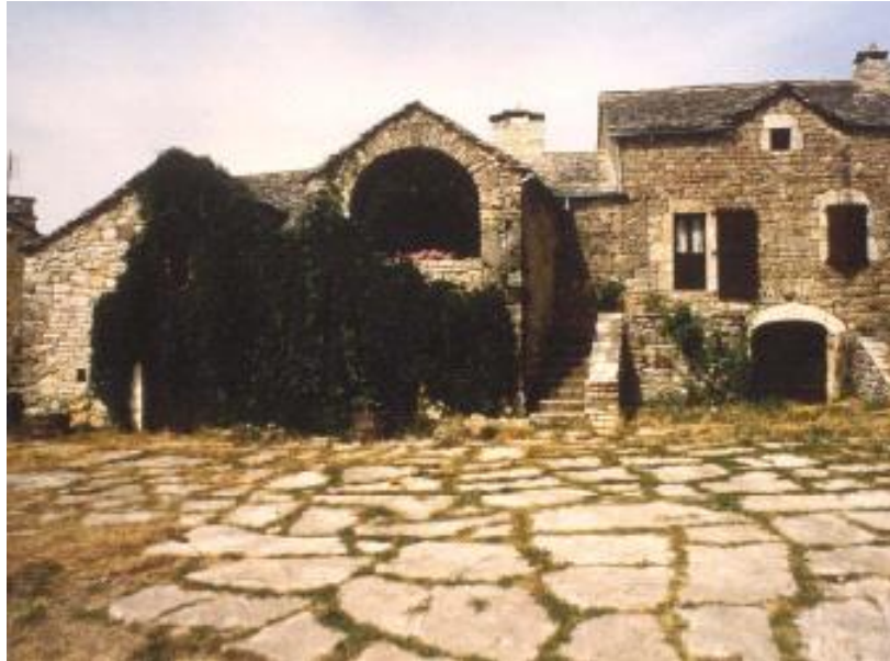
Figure 1: House, Built of stone laid in mud mortar with paving stone yard of stones in mud mortar. Photo: CRATerre/EAG.
