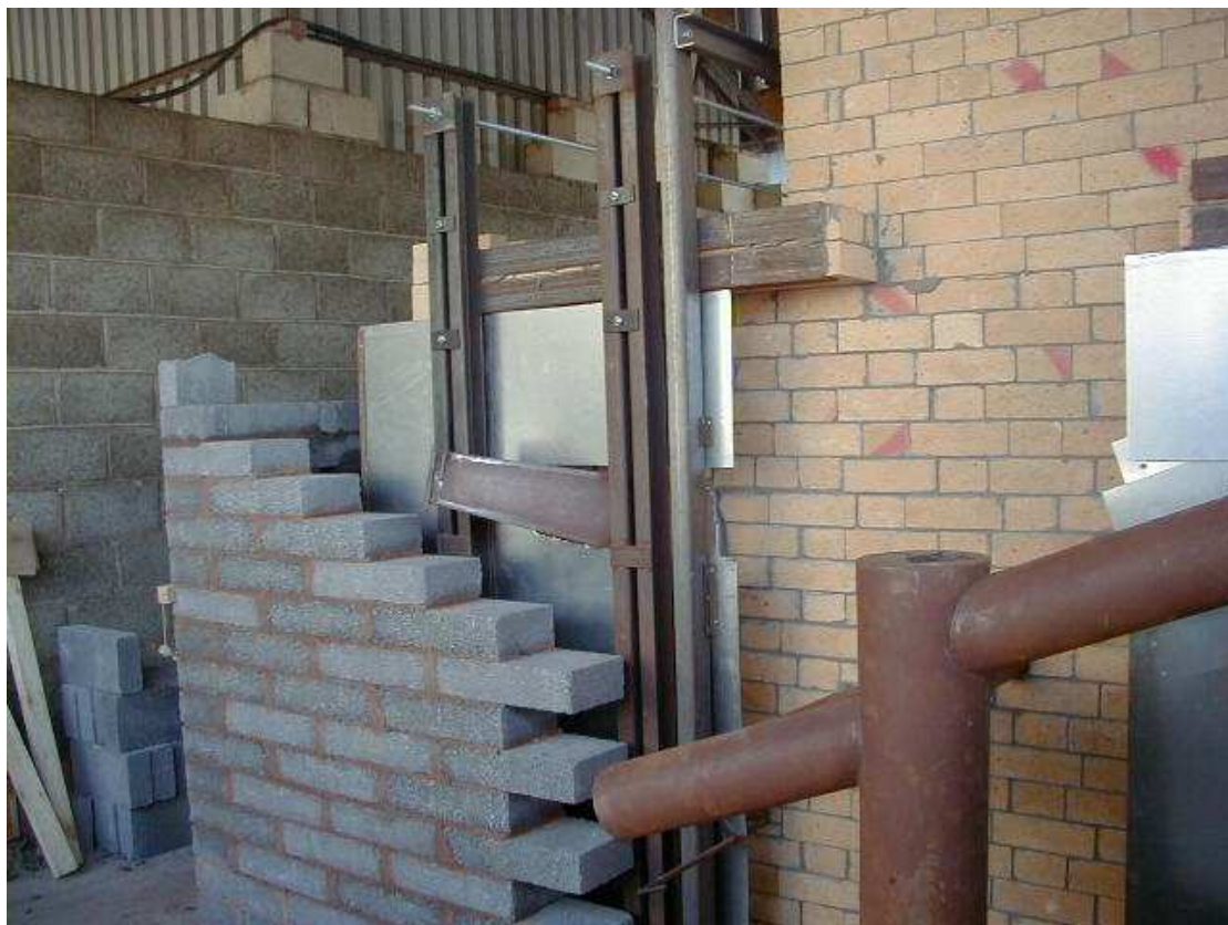
Figure 3.18: Outer wall construction
