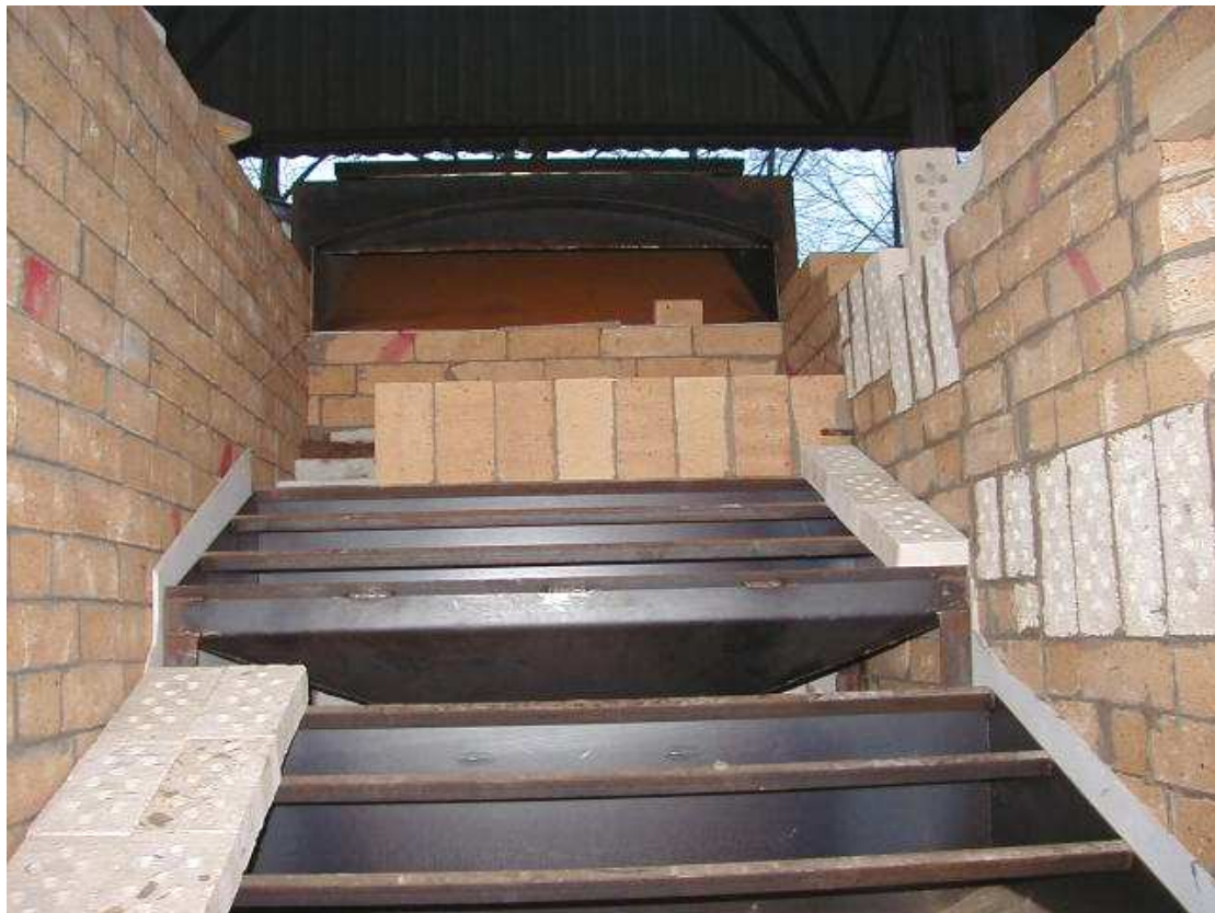
Figure 3.5: Perforated refractory bricks being laid on plenum/grates
