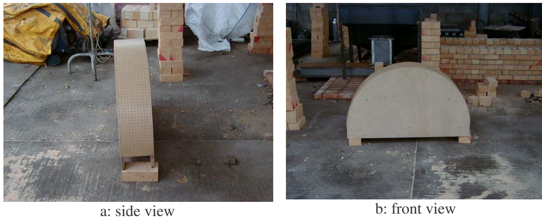
Figure 2.3: Form for access arch
