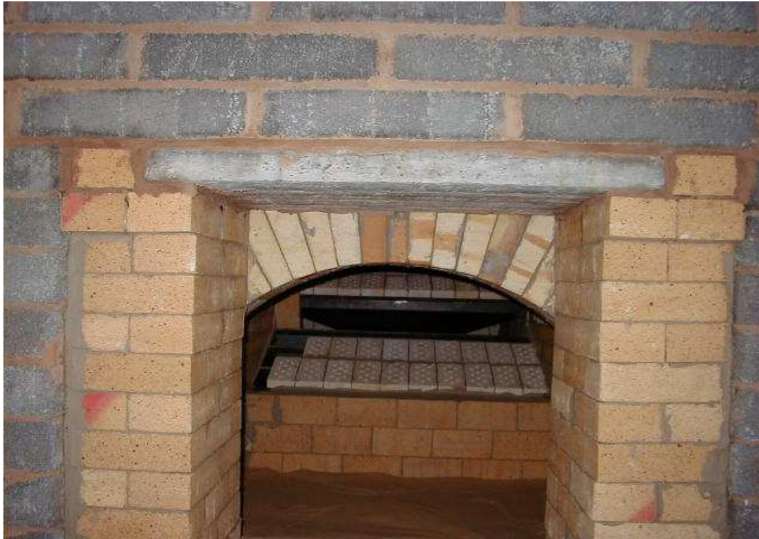
Figure 3.19: Access tunnel from outer wall to combustion chamber access arch (ash-end)
