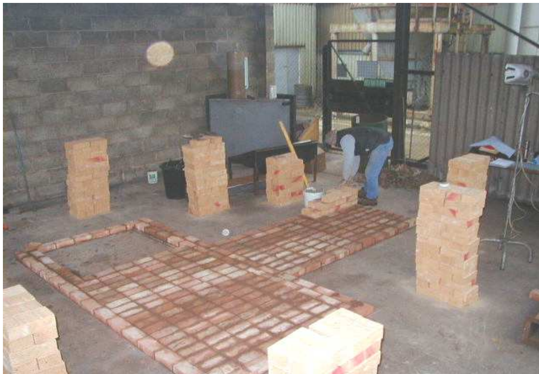
Figure 3.3: Laying refractory bricks (from stack end)
