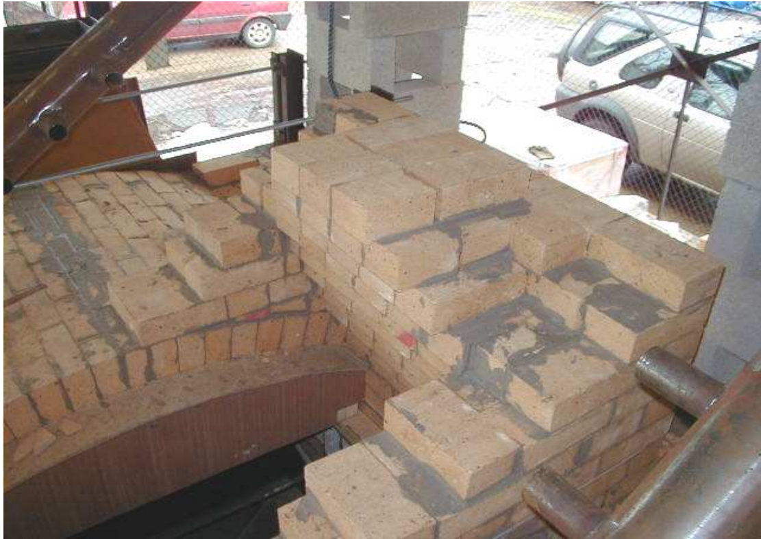
Figure 3.13: Cross connector built on top of primary chamber roof-arch - showing corbelled wall under construction and secondary-air tubes (view from ash end)
