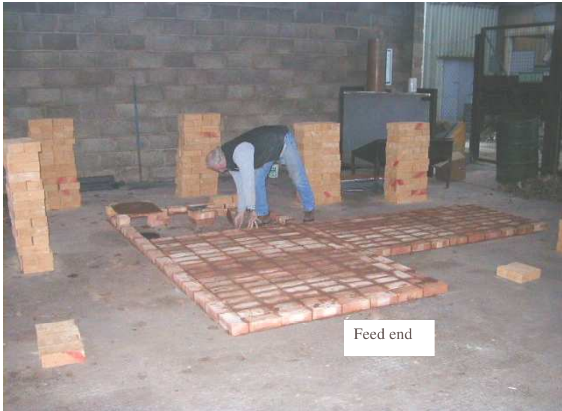
Figure 3.2: Laying LCI floor
