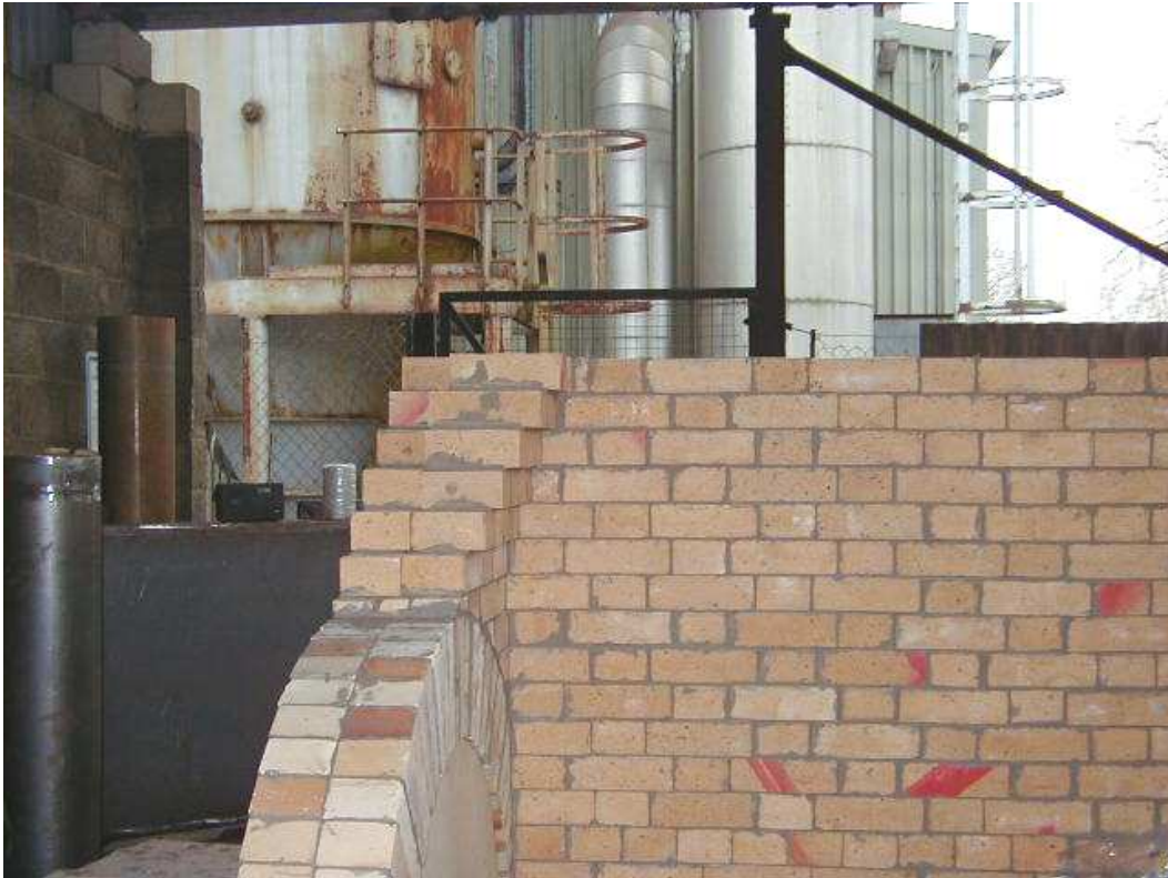
Figure 3.8: Corbelled wall above access arch on Ash End wall of the primary chamber
