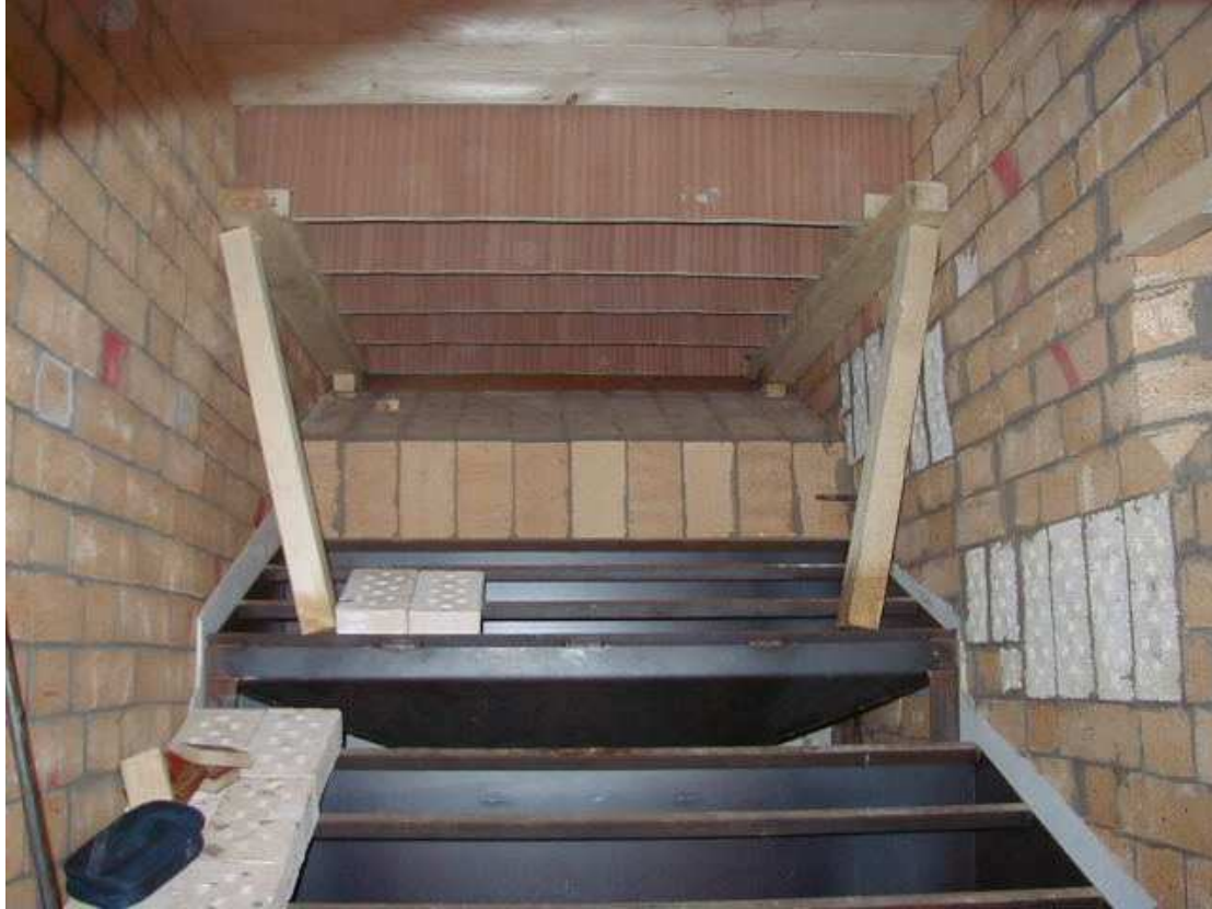
Figure 3.11: Arch form supported by wooden posts
