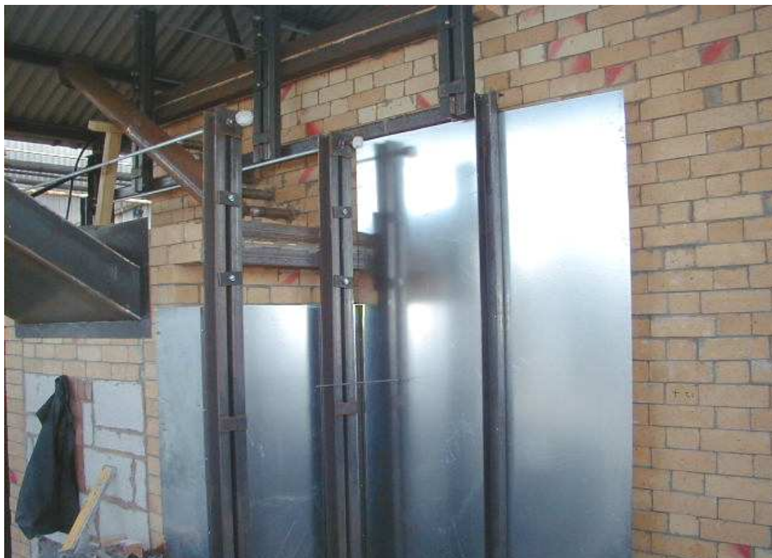
Figure 3.17: Sheet steel retaining wall under construction
