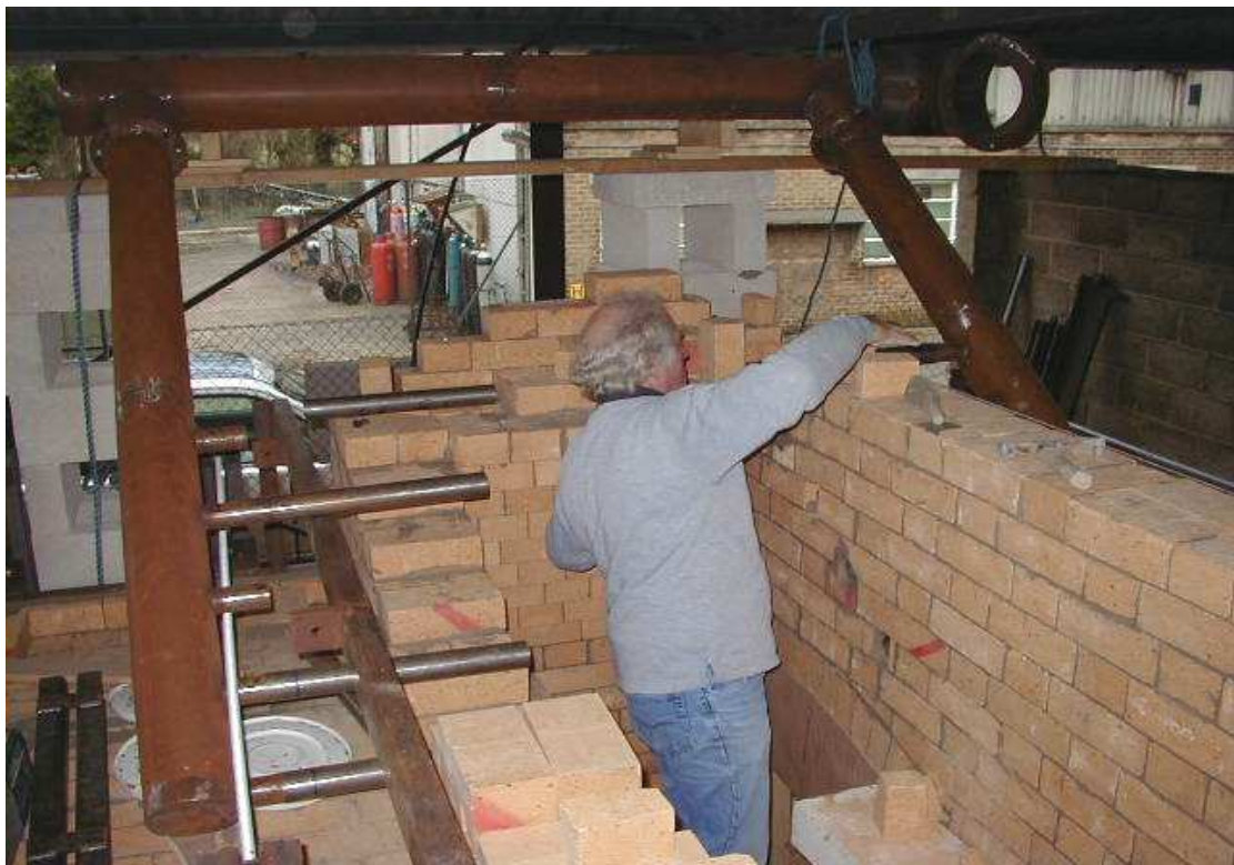
Figure 3.14: Building up the vertical walls of the cross chamber from the corbelled end
