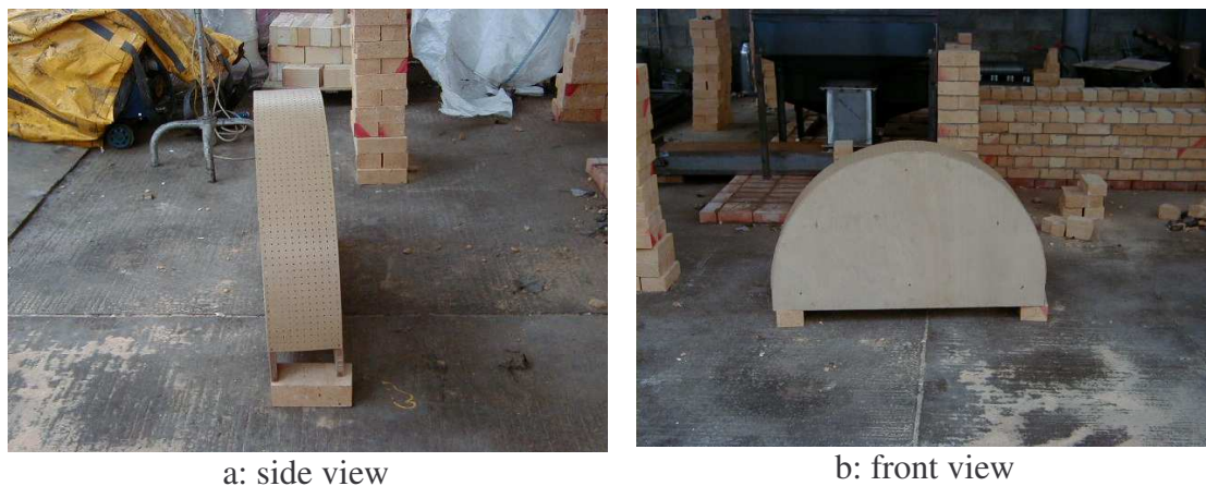
Figure 2.3: Form for access arch
