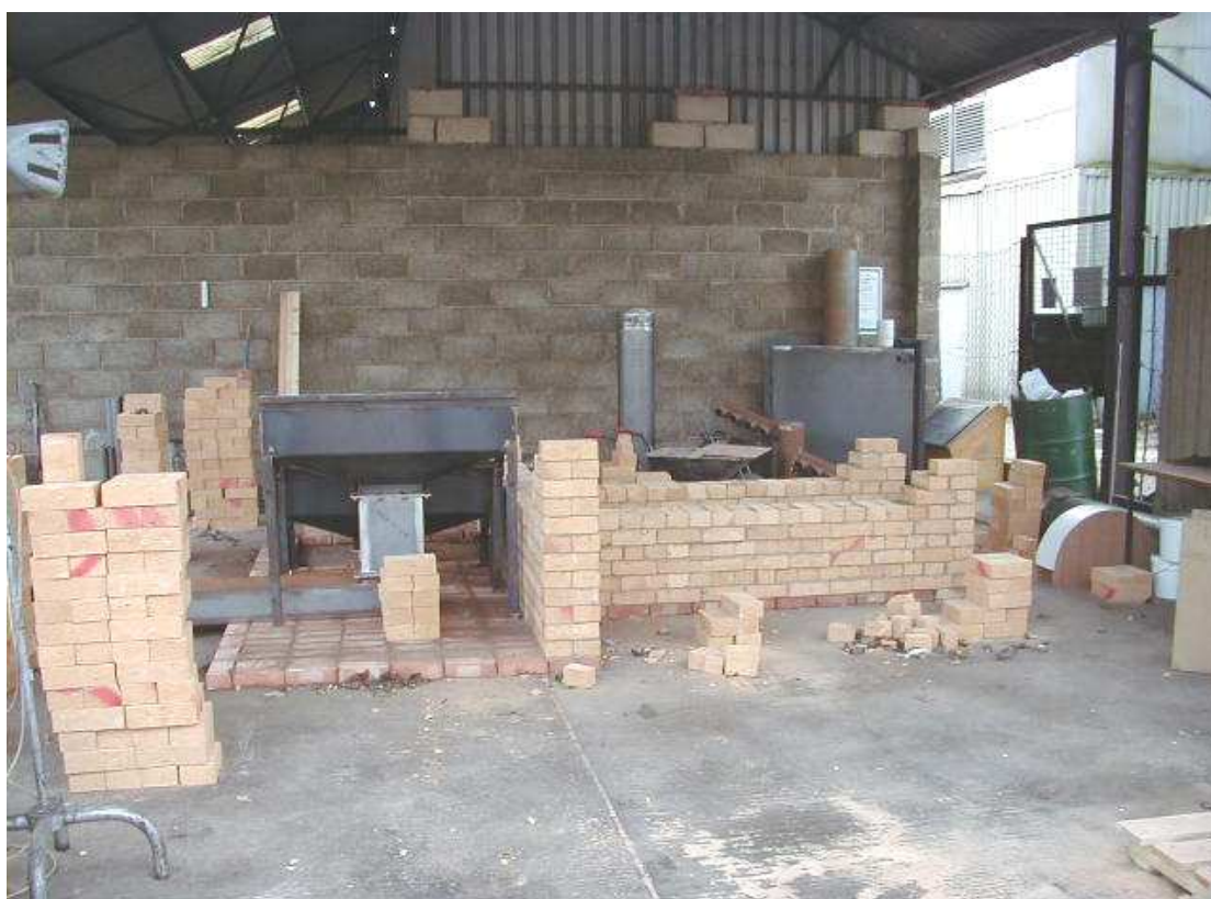
Figure 3.4: Building primary chamber right hand position ( Note: Plenum/grate shown is the prototype design and differs from current design )
