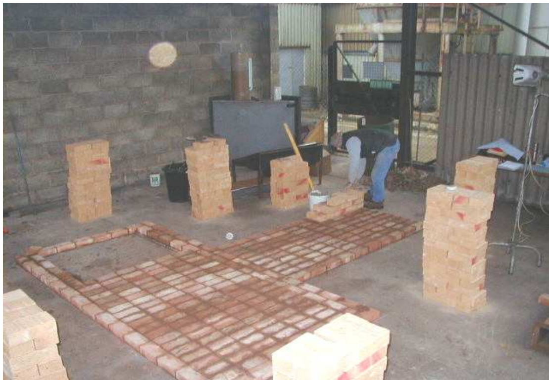
Figure 3.3: Laying refractory bricks (from stack end)
