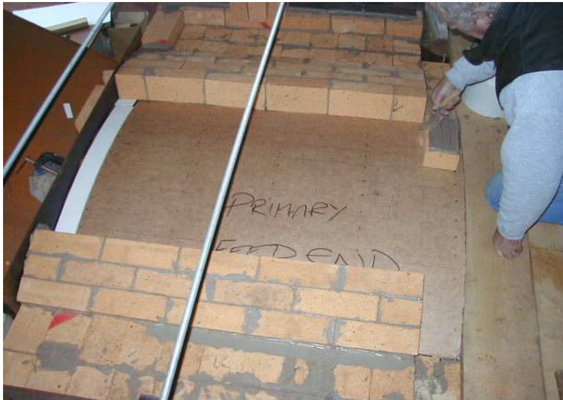
Figure 3.12: Primary chamber arch under construction.
