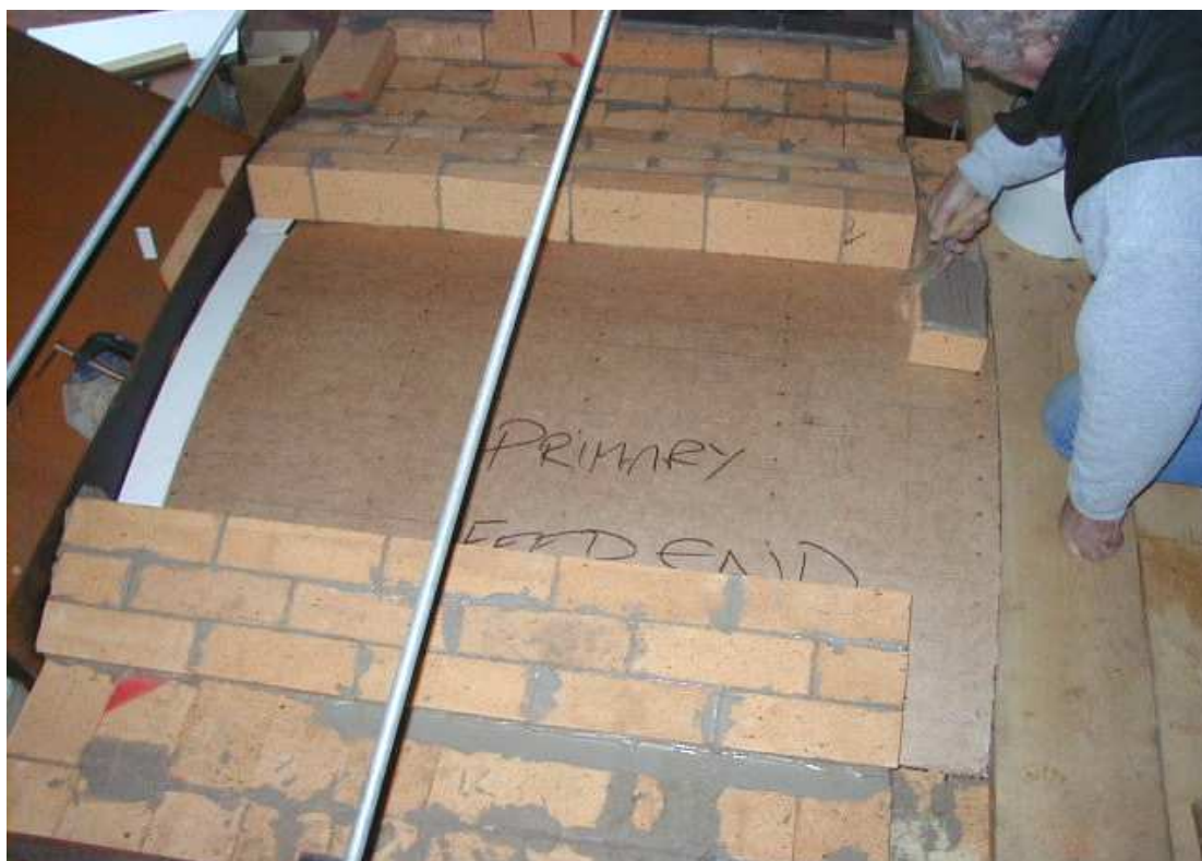
Figure 3.12: Primary chamber arch under construction.
