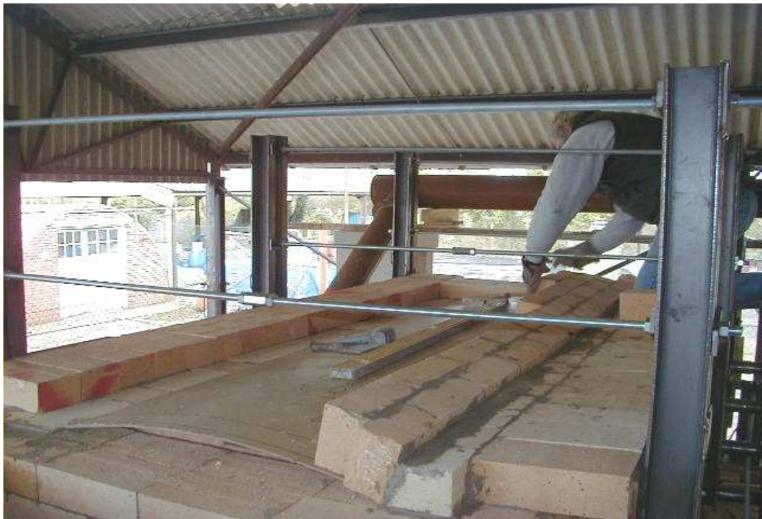
Figure 3.16: Secondary chamber roof-arch under construction – showing arch former and backstays in position
