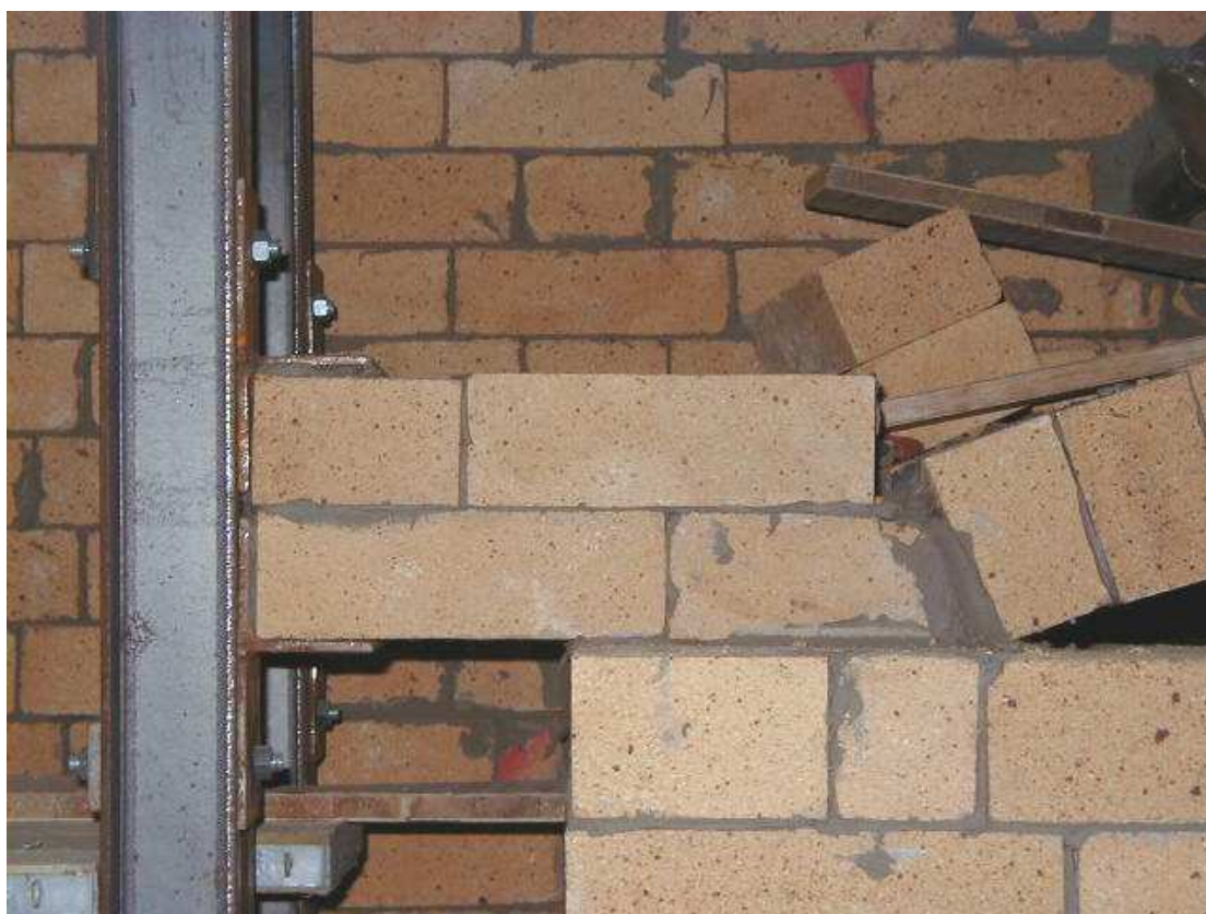
Figure 3.10: Skew-brick and skew-brick rails in position.
