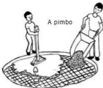
Figure 9: The mesh is covered with more concrete
