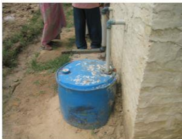
Figure 2: With urine separation one option is to collect the urine so that it can be used as a liquid fertiliser later on. Photo: Practical Action, South Asia.
