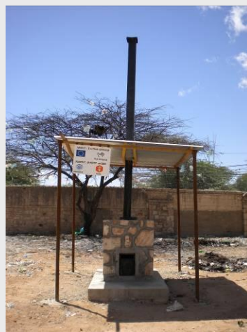
Fig. B.2 – New De Montfort incinerator built at General Group Hospital
