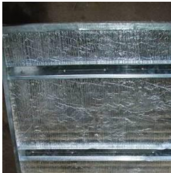
Collector frame mounted to insulated backing frame with spacers
