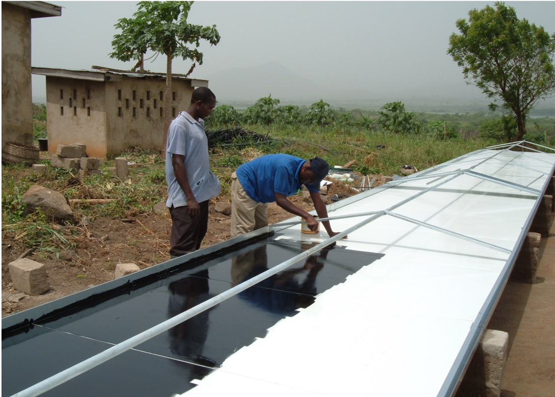
Figure 7: A Hohenheim dryer, Ghana. Black paint being applied to the collector. Photo: Tony Swetman.
