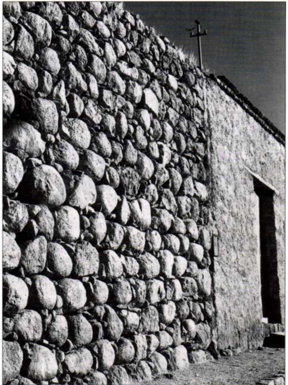
Figure 1: "Granite boulders with snecking in La Rioja Province of Argentina"
